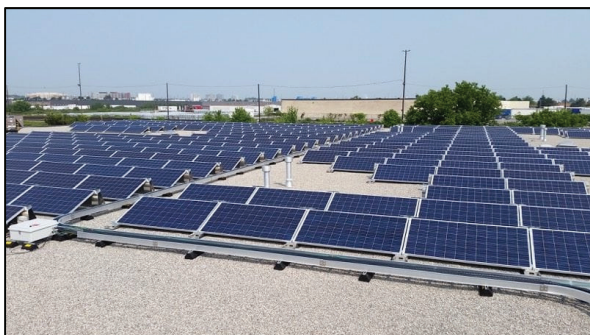
Figure 6: Ballasted racking installation system on flat roof
