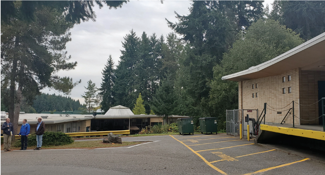
Building Area 1: North
