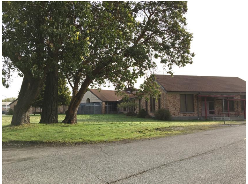
Photo of Building 27 before remodeling.
