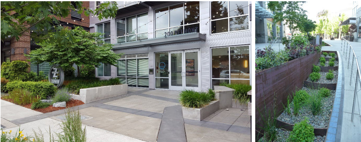
Left image includes a good landscaping example for a major building entrance, with a variety of plant materials and hardscape elements to create an inviting entry. The right image includes playful rain garden landscaping within a public place.
