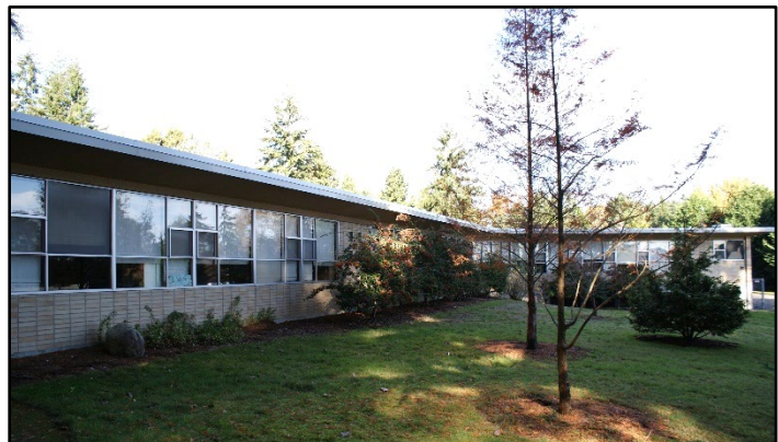
Figure 2.6 Existing nursing facility
