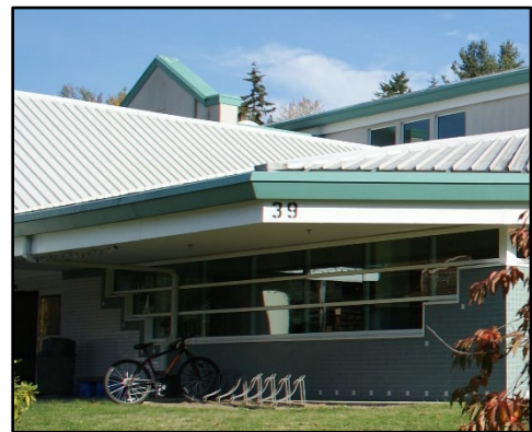
Figure 5.16 Building number signage on the Kitchen building
