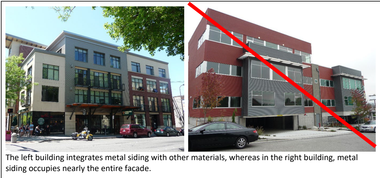
Figure 5.13 Metal Siding Examples
