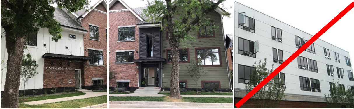
Figure 5.14 Cementitious Wall Board Examples
