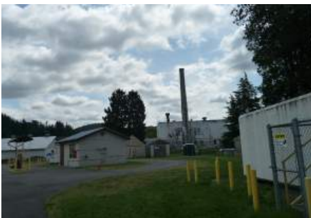
CMO: Northeast campus maintenance buildings
