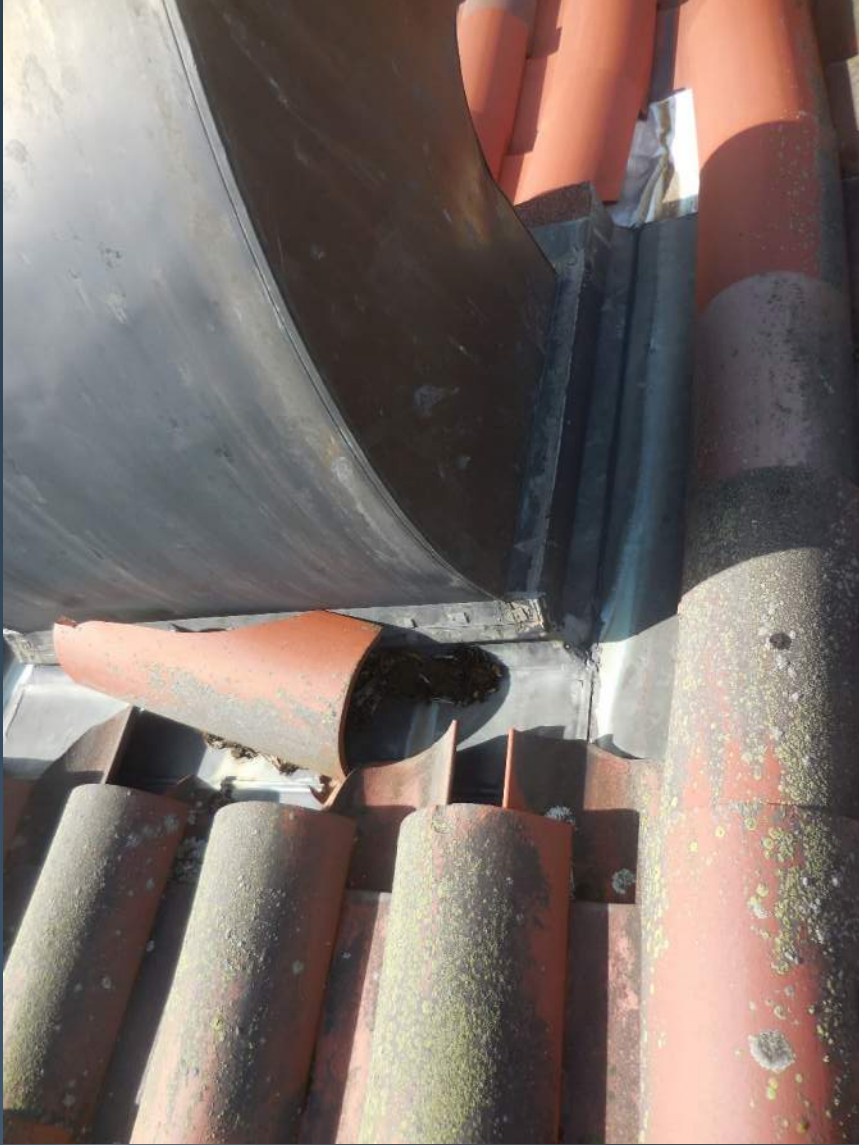
Photos of flashing conditions at typical HVAC Hood.
