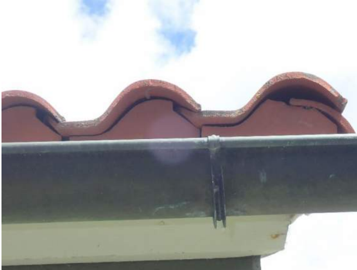
Photo No. 10 - Interlocking Clay Roof Tile Profile
