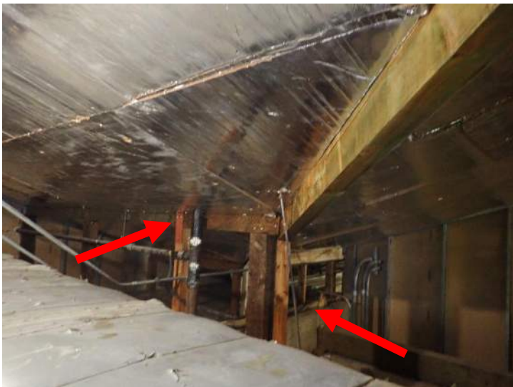
Photo No. 35 - Evidence of Water-Staining at Valleys
