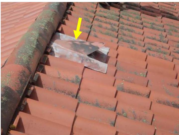
Photo No. 27 - Example gable vent at north end roof area
