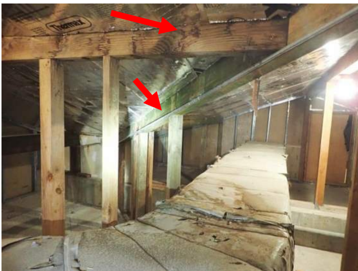
Photo No. 36 - Evidence of Water-Staining at Valleys
