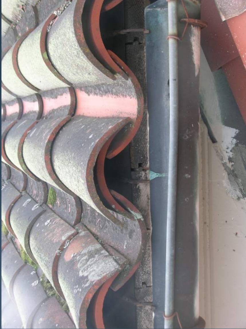
Photos of conditions at downslope eave edge flashings.
