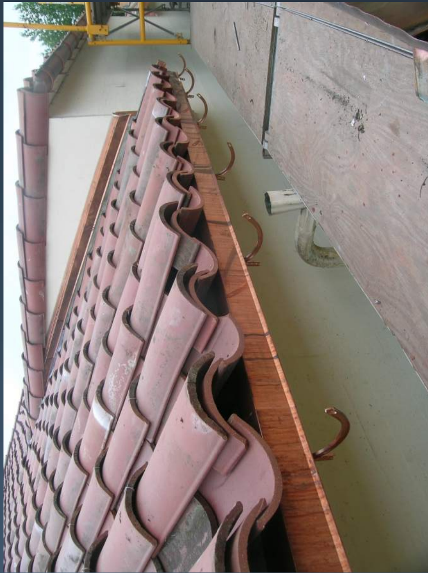
Gymnasium/Office Wing downslope eave edge at retrofit copper gutters.
