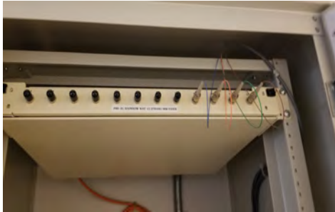
Existing Fiber Patching.
