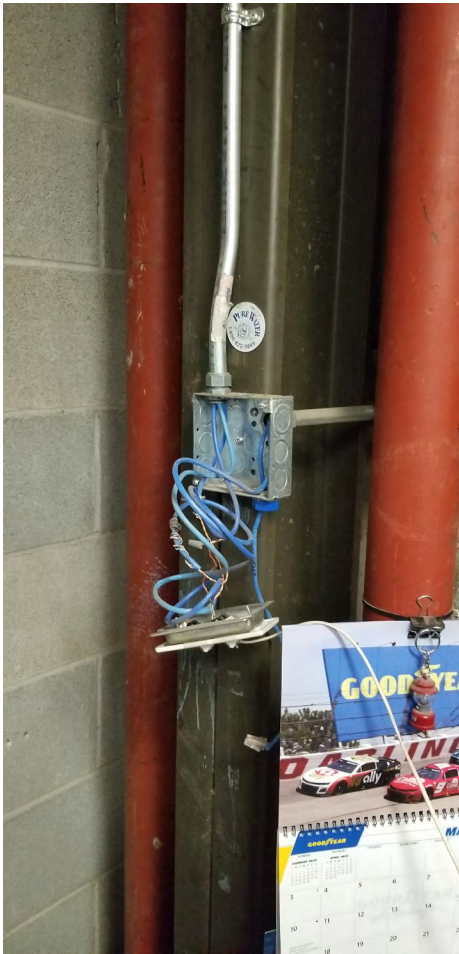
Damaged Data Outlet.
