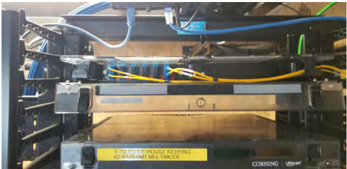
Existing SM Rack Mount Fiber Cabinet.
