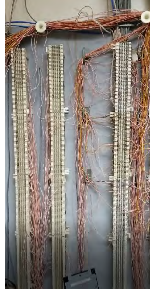
Existing 66 & 110-Blocks for Voice Patching.
