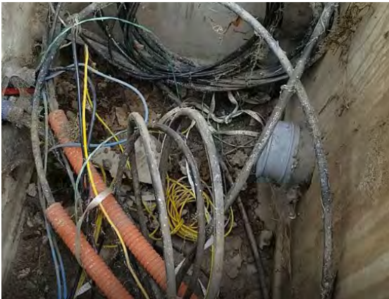
Existing Interbuilding Backbone Cabling.
