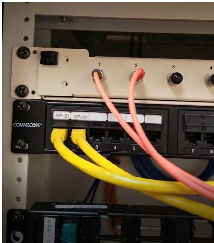
Existing Fiber and Data Patching.
