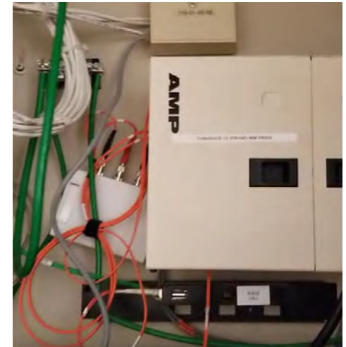
Existing Fiber Patching.
