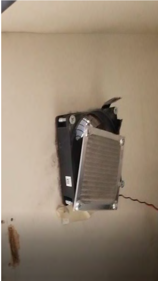
Existing Cabinet Cooling Fan.
