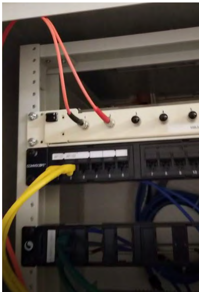
Existing Fiber & Data Patching.
