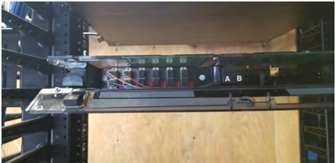
Existing MM Rack Mount Fiber Cabinet.
