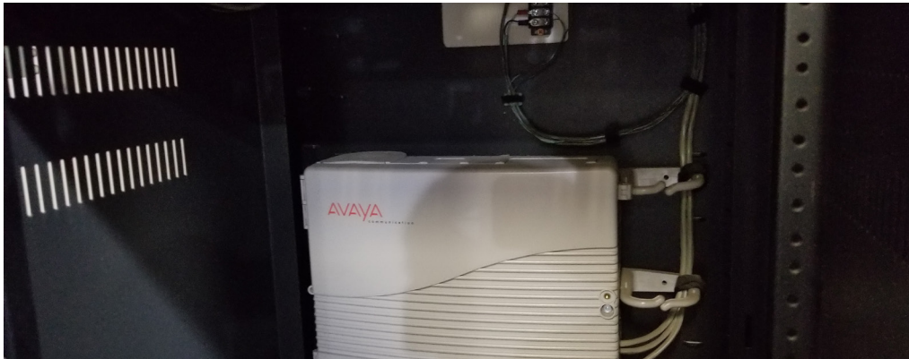
Existing Building Entrance Protection.
