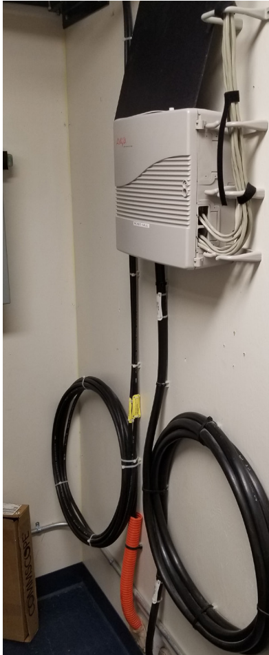
Existing Building Entrance Protection.
