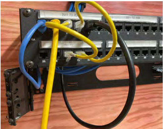
Existing Data Patching.
