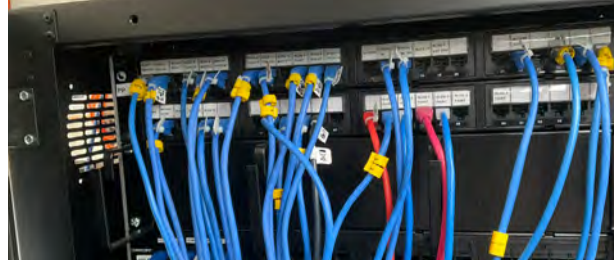
Existing Data Patching.
