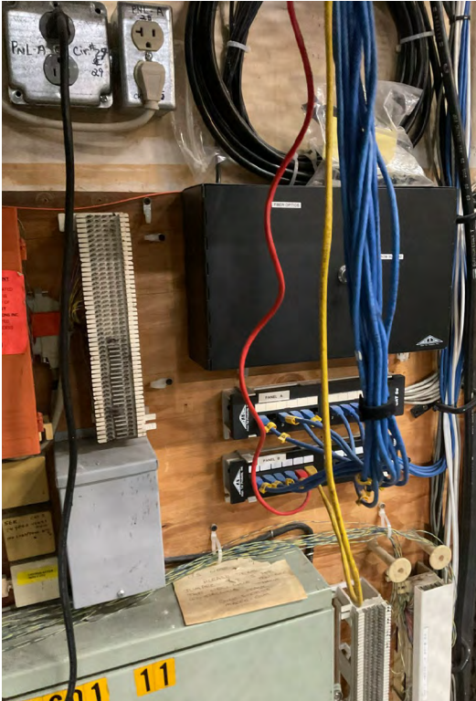
Existing Data Patching.
