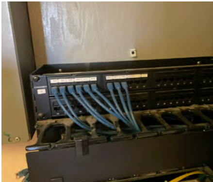
Existing Data Patching.
