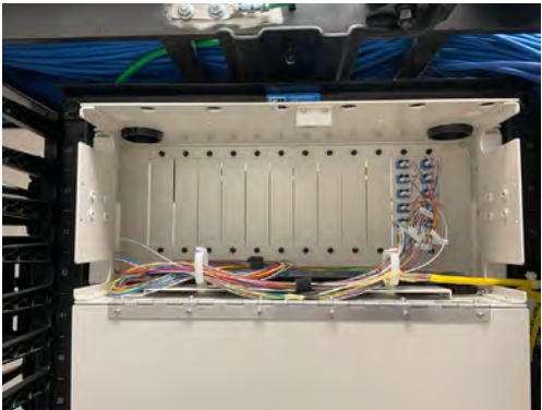
Existing Backbone SM OFC.
