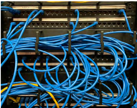
Existing Data Patching.
