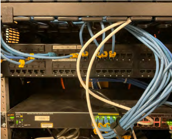
Existing Data Patching.
