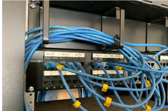
Existing Data Patching.
