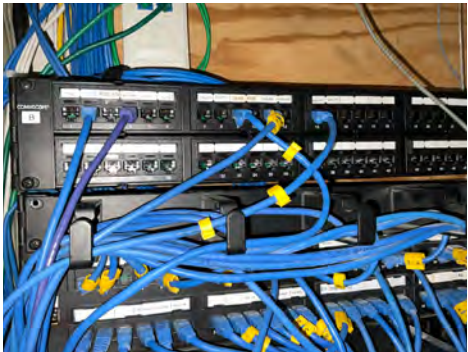
Existing Data Patching.
