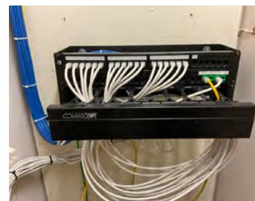
Existing Data Patching.
