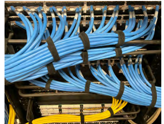
Existing Data Patching.
