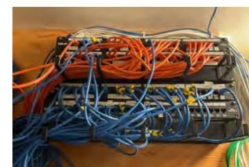
Existing Data Patching.
