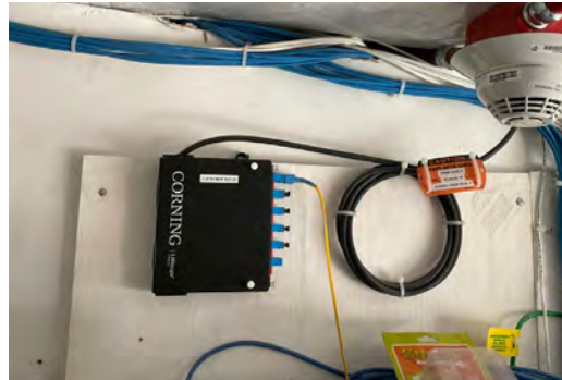
Existing Backbone OFC.
