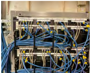
Existing Data Patching.
