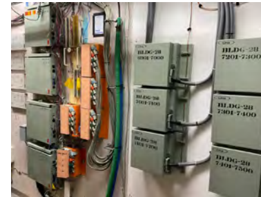
Existing Entrance Protections.
