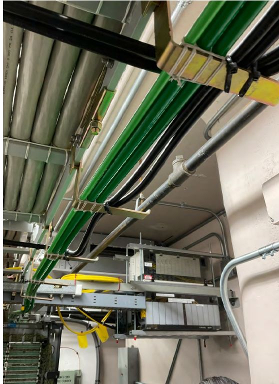
Existing Cable Supports.
