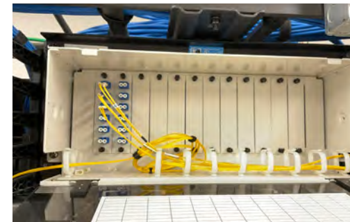
Existing Backbone SM OFC.
