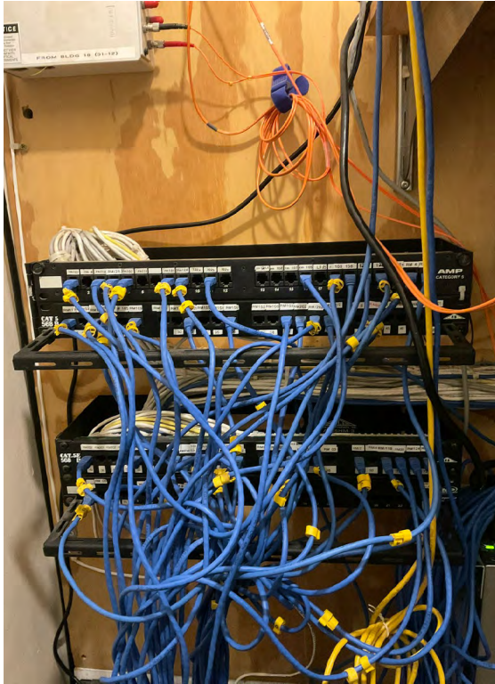
Existing Data Patching.
