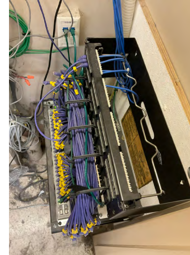
Existing Data Patching.
