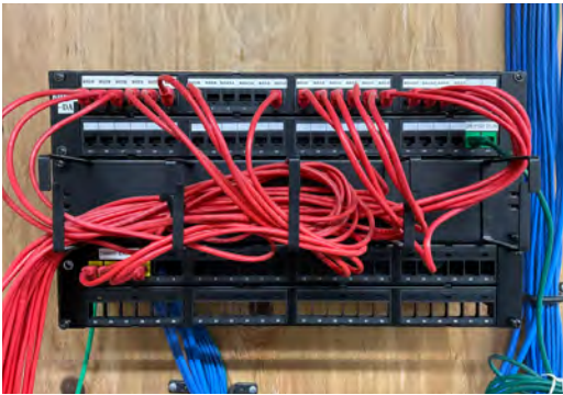
Existing Data Patching.
