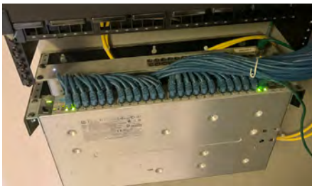
Existing Wall Mounted Bracket.
