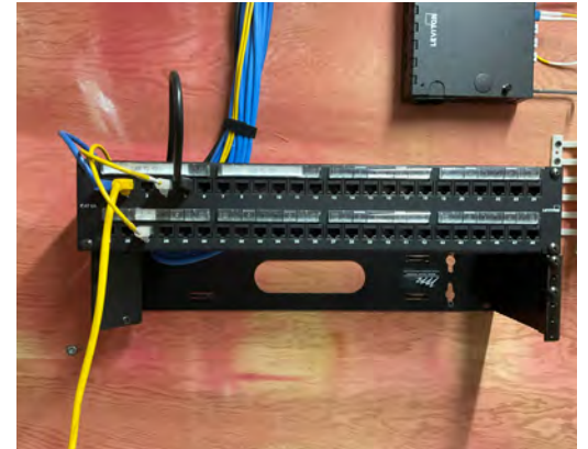
Existing Data Patching.
