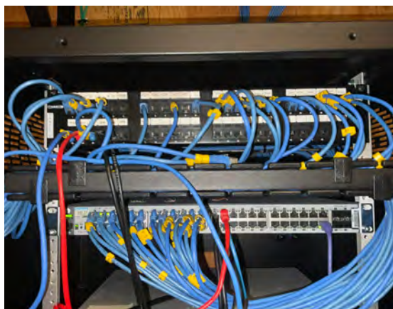
Existing Data Patching.
