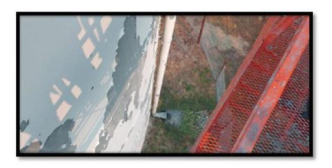
The paint is flaking off exterior of the water tower.
