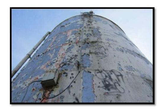
The paint is flaking off exterior of the water tower.
