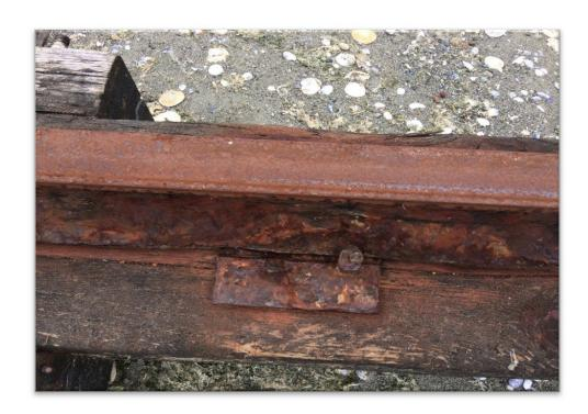
The fasteners have corroded and are failing.
