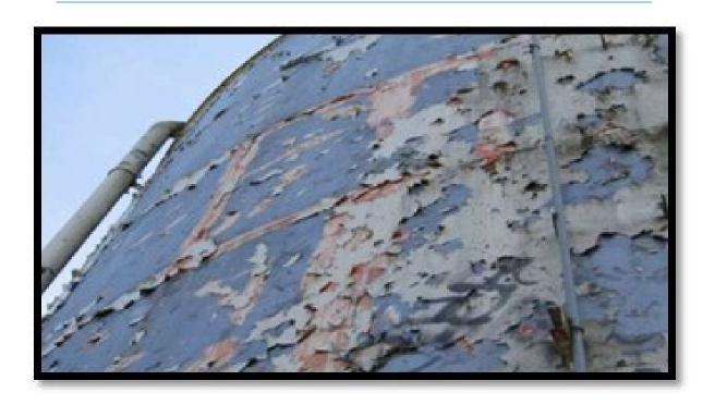
The paint is flaking off exterior of the water tower.
