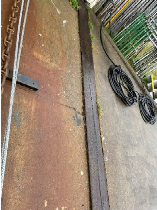
Photo 128: Timber rail beam (A) North of bulkhead
