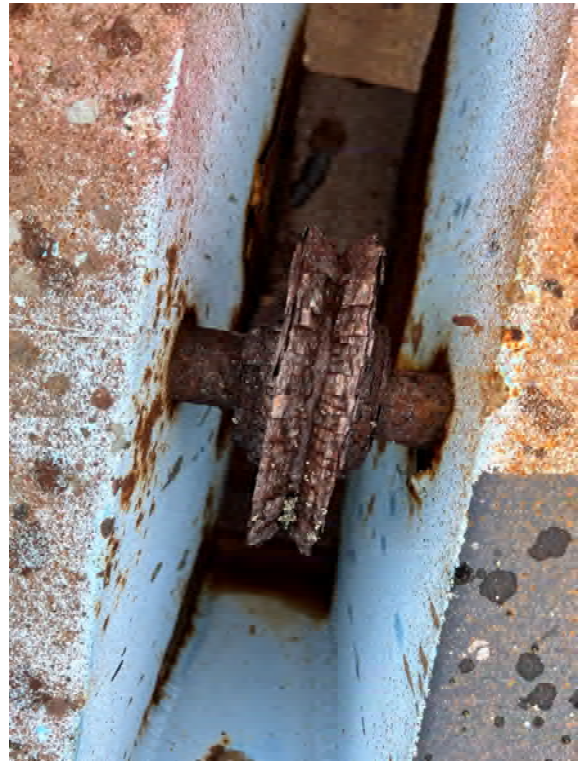
Photo 192: Bilge block pulley
