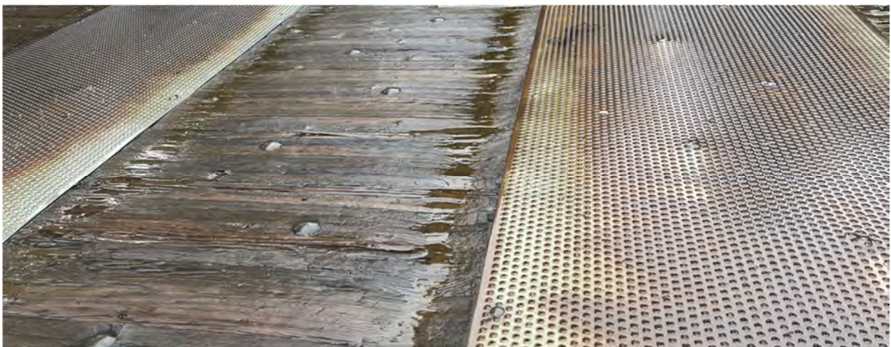
Photo 103: Timber deck is rutting
