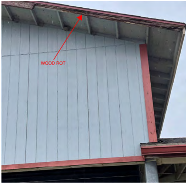
Photo 79: Wood rot on Fascia board
