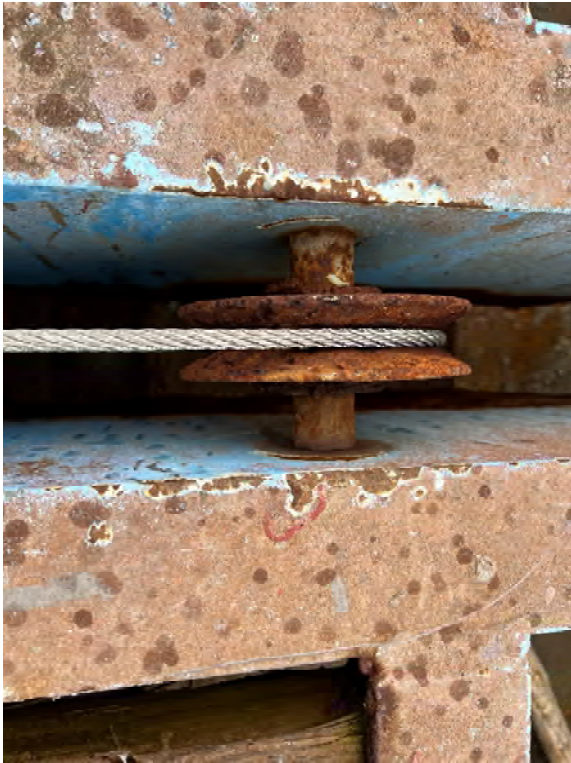
Photo 191: Bilge block pulley
