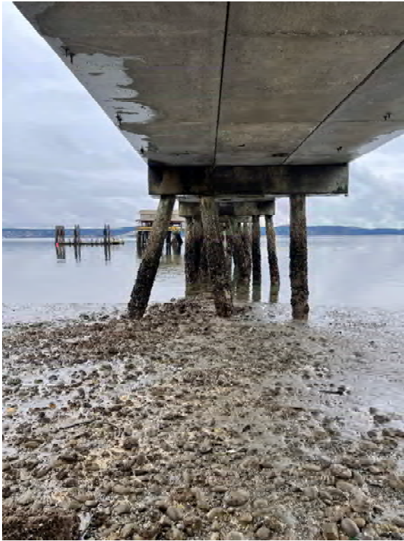
Photo 71: Concrete spalling below trestle
