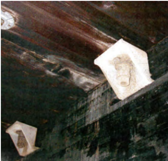
Photo 83: Loose timber deck hold down bolts
