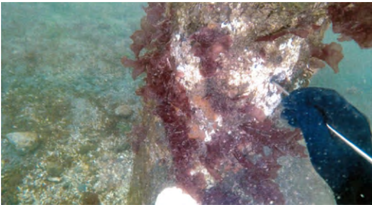
Photo 12: Pile 3B two marine borer entries (MBE)
