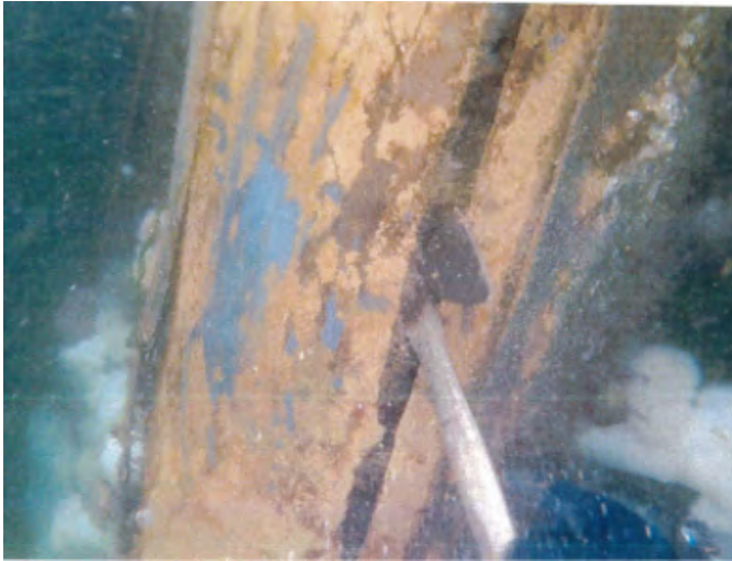
Photo 43: SP1-A holed through
