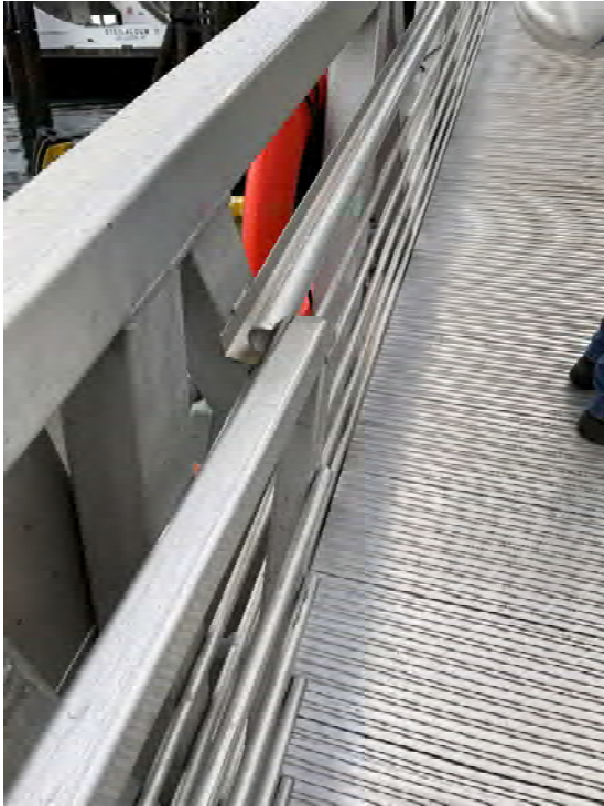
Photo 21: Loading ramp handrail with sharp edge
