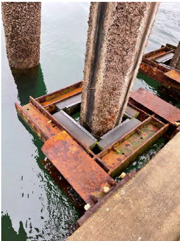
Photo 27: Pile collar with bent angle
