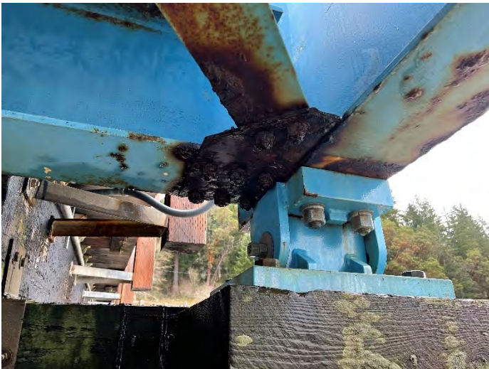
Photo 97: Heavy surface corrosion on fasteners
