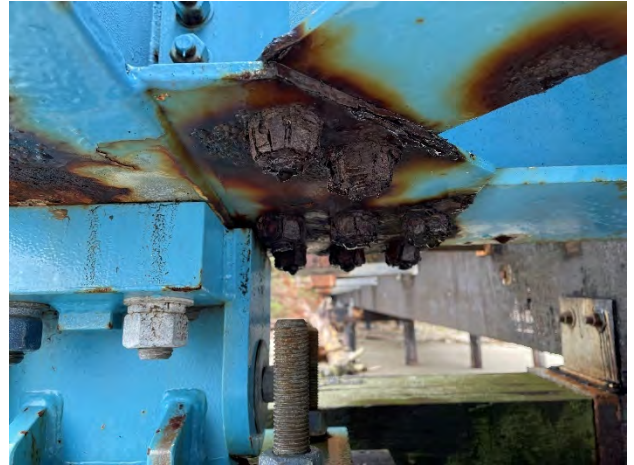
Photo 100: Heavily corroded and delaminating nuts
