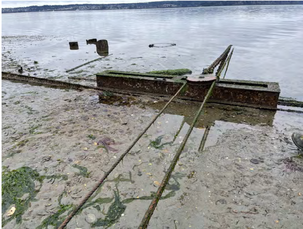
Photo 154: Anchor system at Southern end of track
