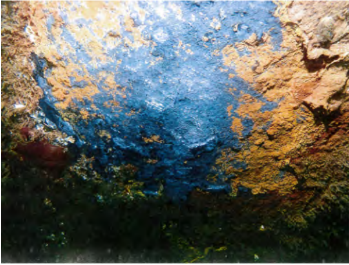
Photo 33: SP3B surface corrosion and section loss
