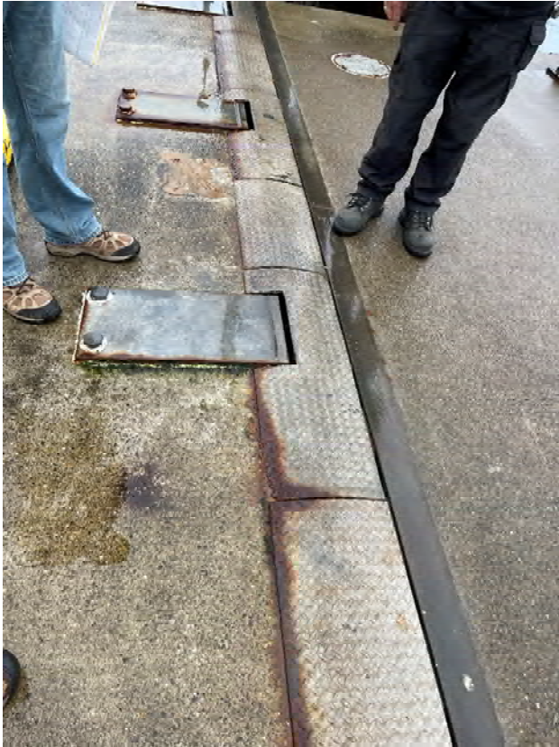
Photo 59: Surface corrosion on cover plate
