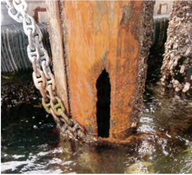
Photo 39: SP4-A holed through
