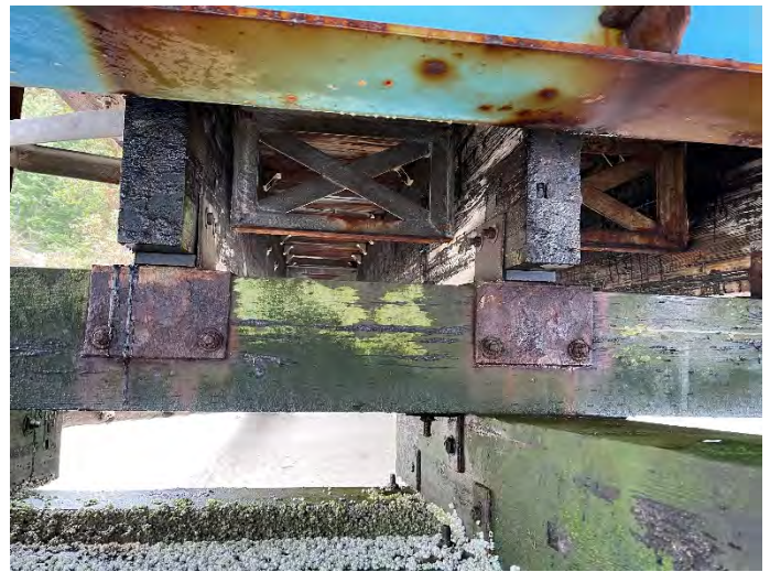
Photo 98: Heavy surface corrosion on girder brackets
