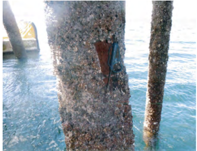
Photo 11: Pile 8.9A Rot cavity (2019)
