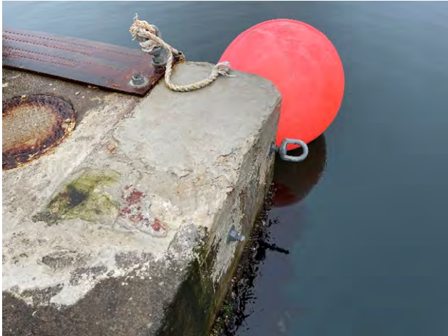
Photo 51: Fender removed and concrete float patched
