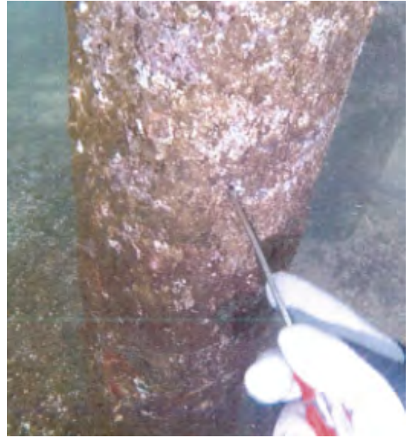
Photo 82: Pile 4A Marine borer entry
