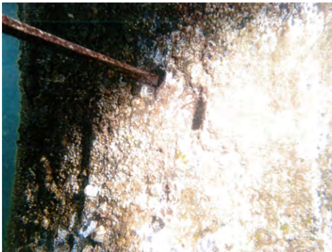
Photo 12: Pile 3B two marine borer entries (MBE)
