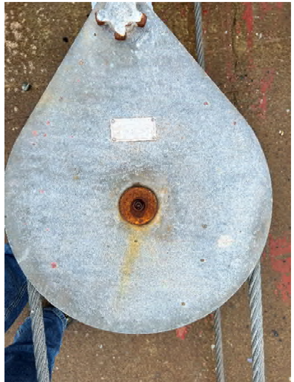
Photo 175: Snatch block on South end of cradle
