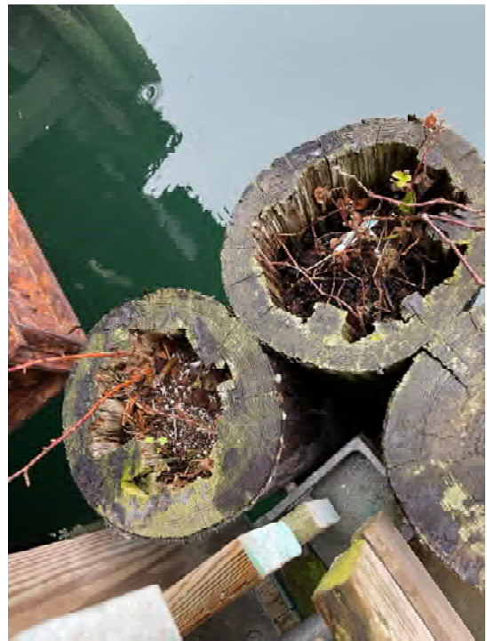
Photo 78: Piles F2A,B,C rot at top of piles
