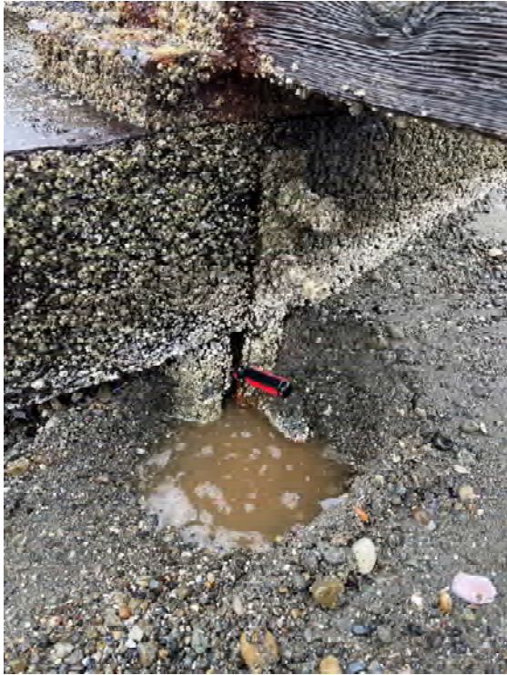
Photo 146: Pile 10B, hollowing around pile cap fastener
