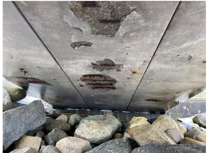
Photo 72: Concrete spalling below trestle
