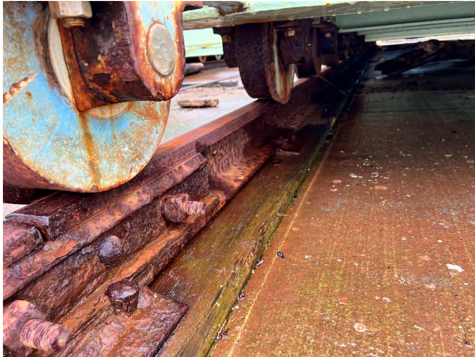
Photo 196: Cradle wheels and rails
