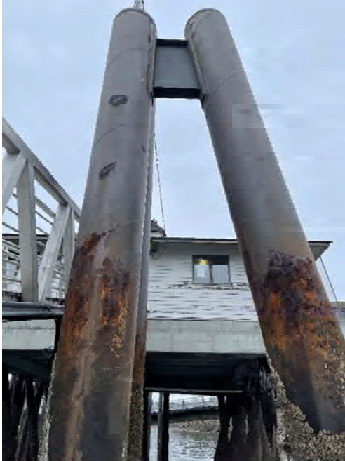
Photo 29: Plumb pile and batter pile
