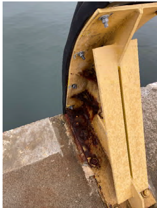
Photo 24: Fender with surface corrosion
