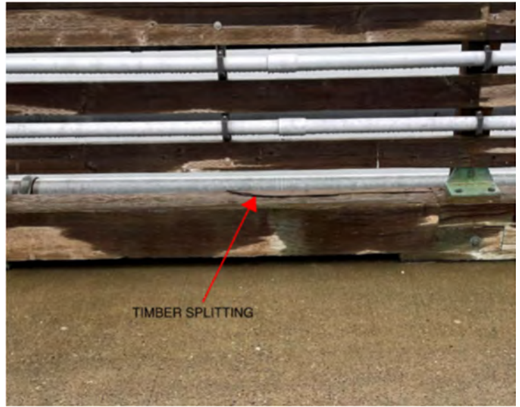
Photo 80: Timber curbing splitting on trestle
