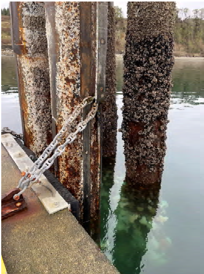
Photo 57: SP3 chain catching on UHMW rub rails
