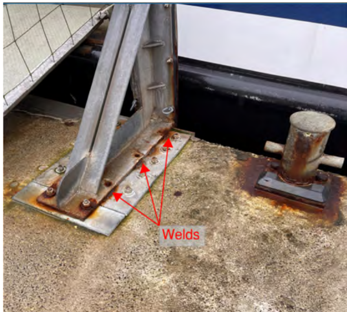
Photo 49: Missing fasteners on fender, secured by welds
