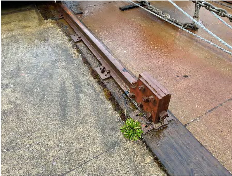
Photo 126 : Surface corrosion on rail North of bulkhead
