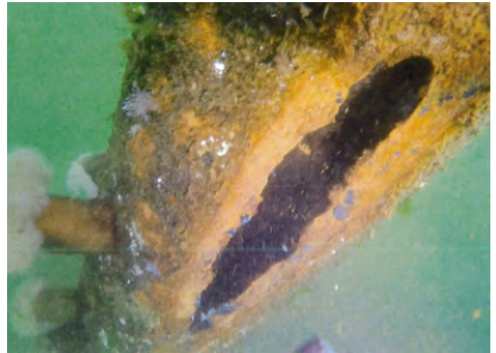
Photo 119: Pile L, 3" W x 24" H hole from mechanical abrasion
