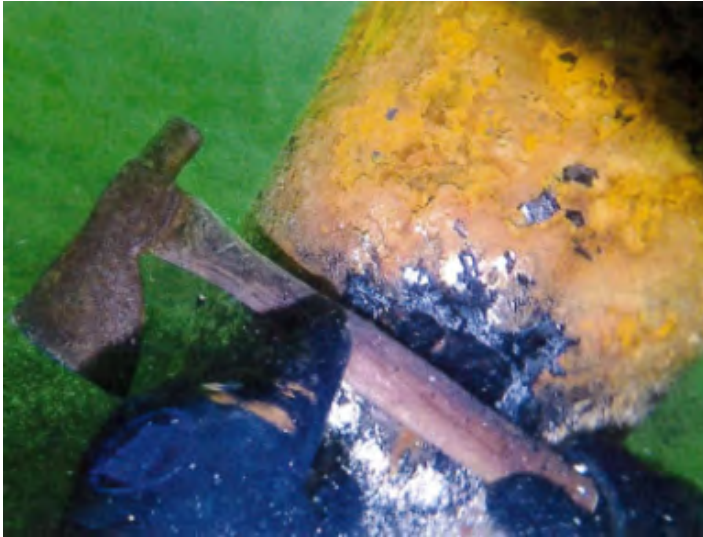
Photo 115A: Pile D, 5" W x 2" H hole
