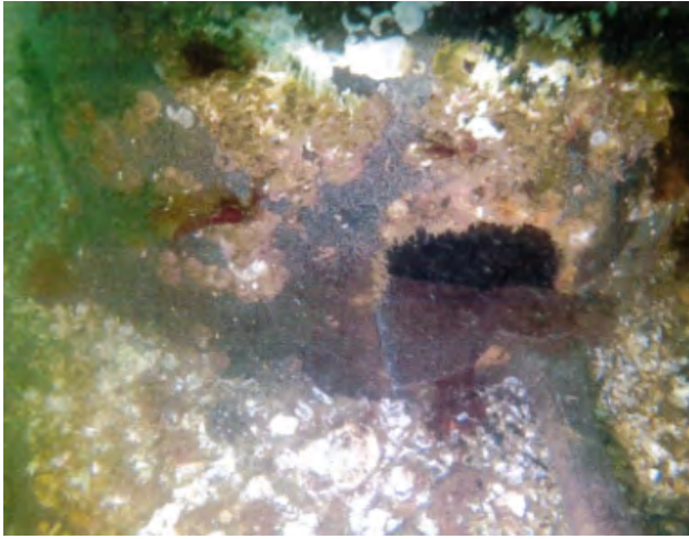
Photo 35: SP1-D holed through
