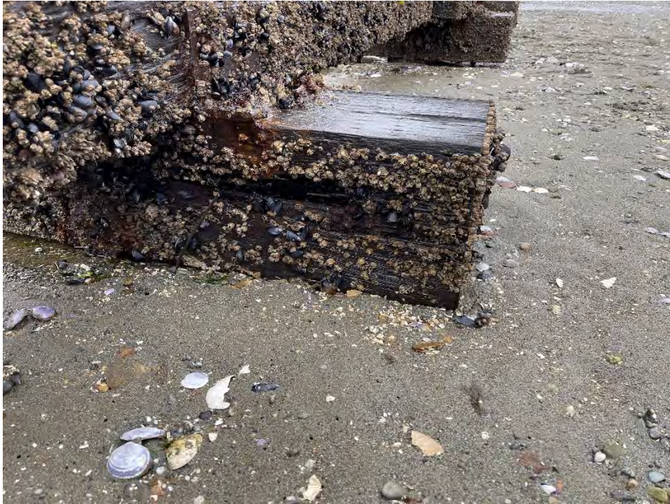
Photo 150: 16 th pile cap with hollowing
