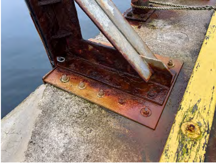
Photo 47: Fender with surface corrosion
