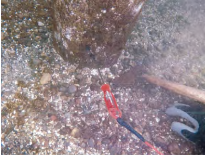
Photo 81: Pile 2C Marine borer entry
