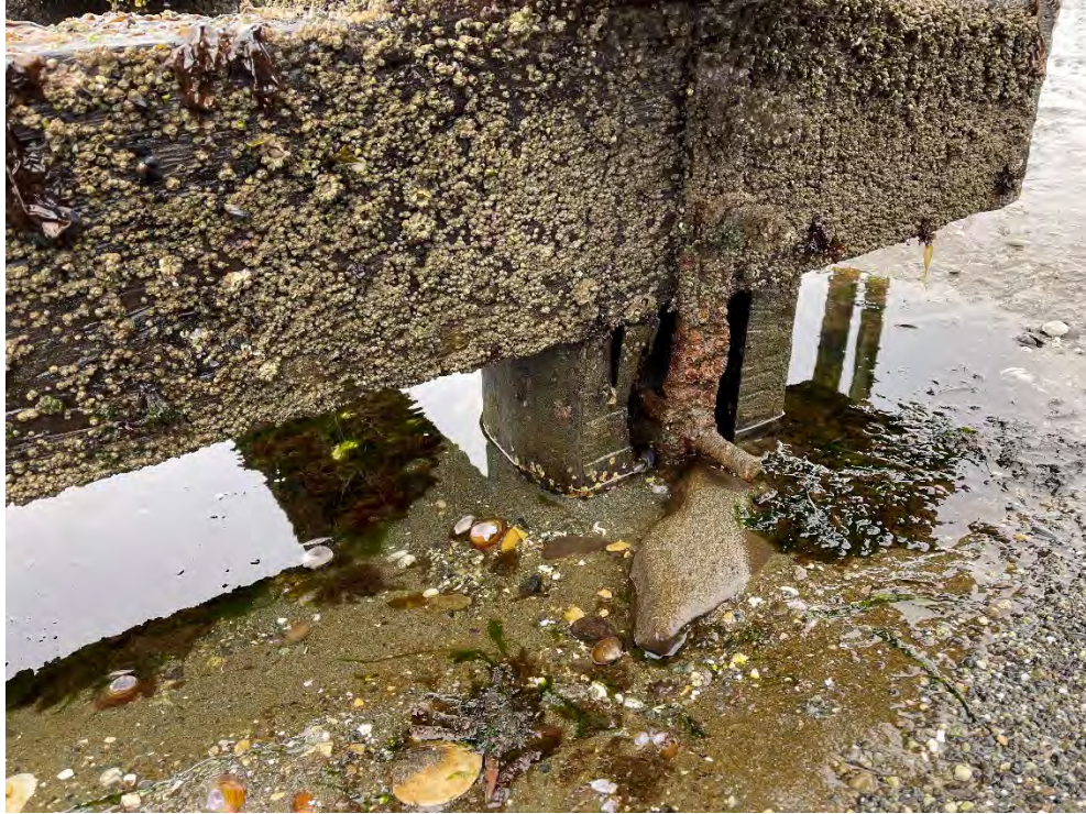
Photo 153: Pile 12A, hollowing around pile cap fastener
