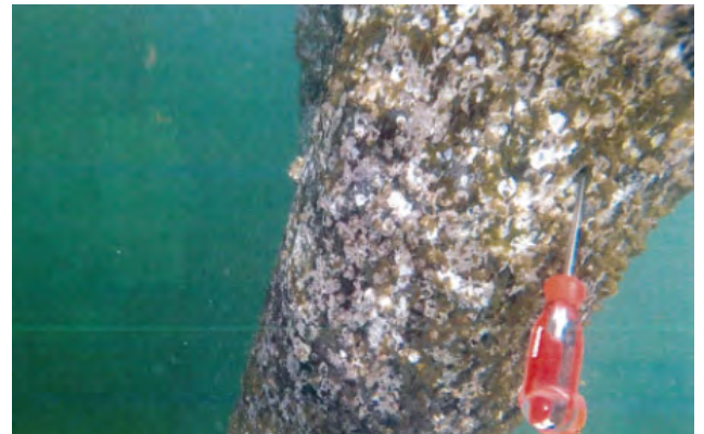
Photo 13: Pile 7.1H marine borer entry (MBE)
