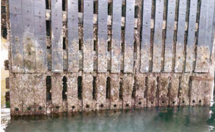
Photo 85: Left wingwall with rot below UHMW sheets
