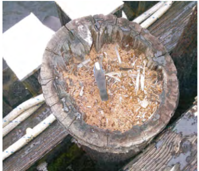
Photo 84: Typical wingwall pile with top rot
