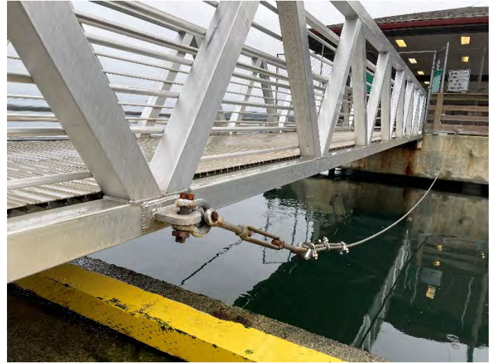
Photo 44: Tie back cable attachment
