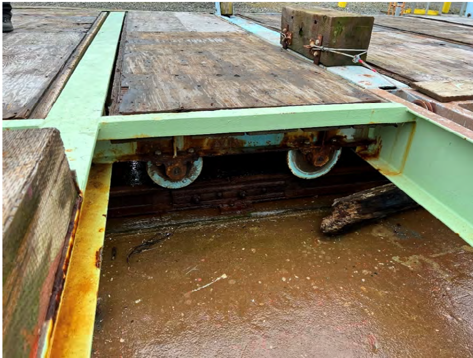
Photo 181: Cradle wheels and decking
