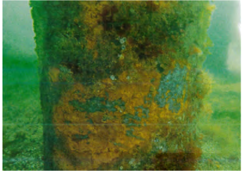
Photo 34: SP4 coating failure and surface corrosion
