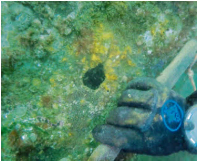
Photo 37: SP3-B holed through
