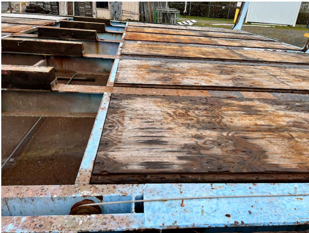
Photo 190: Bilge block pulley
