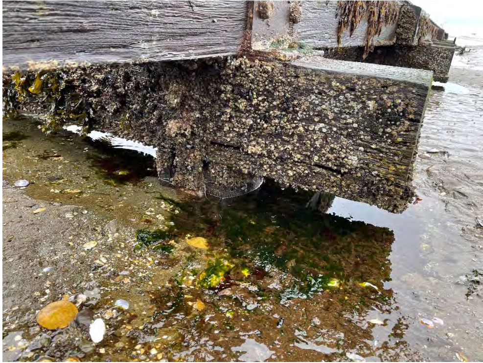
Photo 152: Pile 8B, early stages of hollowing
