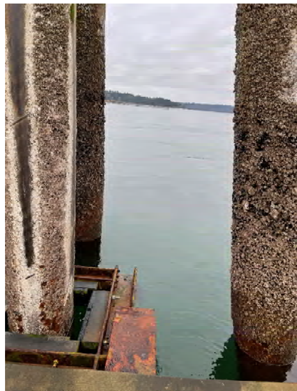
Photo 28: Pile collar with bent angle from batter pile
