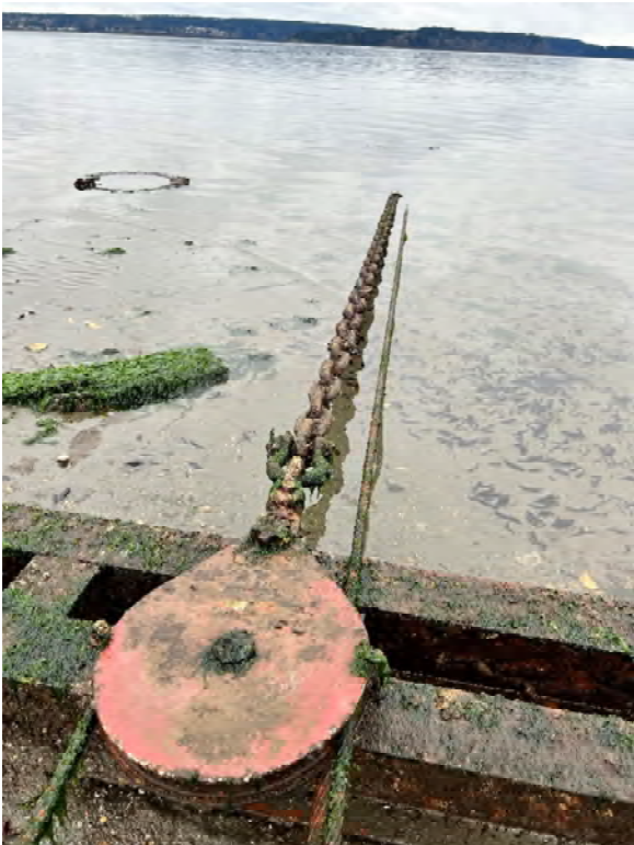
Photo 174: Snatch block on South end of rail system
