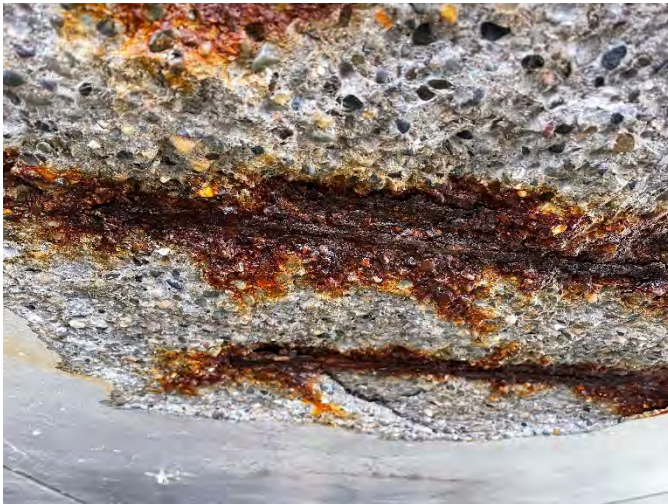
Photo 73: Exposed reinforcement from concrete spalling
