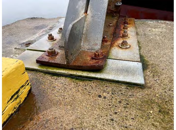
Photo 48: Bent fender with surface corrosion
