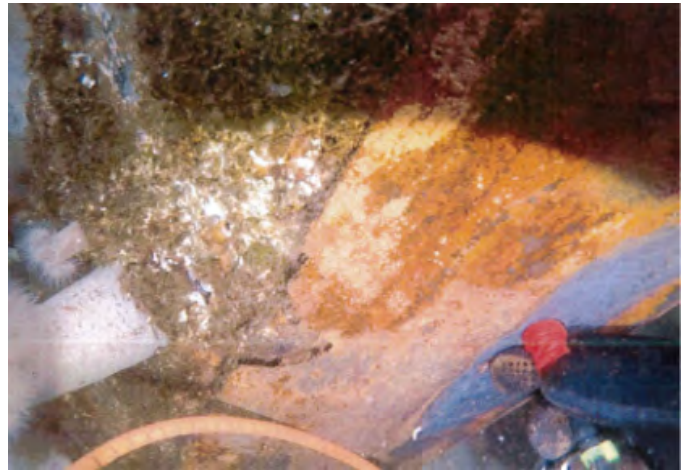
Photo 36: SP2-A heavy corrosion and section loss
