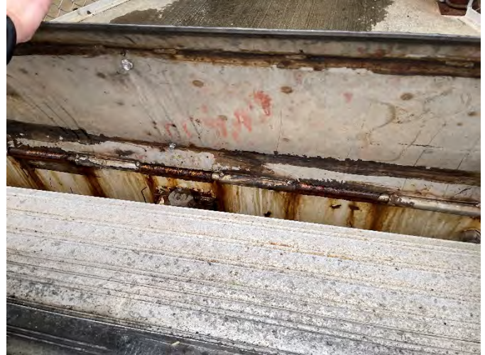
Photo 60: Surface corrosion on connections between floats
