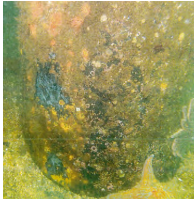
Photo 42: SP4-B typical coating failure and surface corrosion
