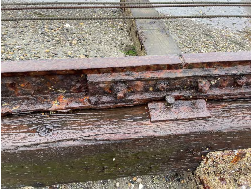
Photo 138: Rail splice plate with heavy surface corrosion
