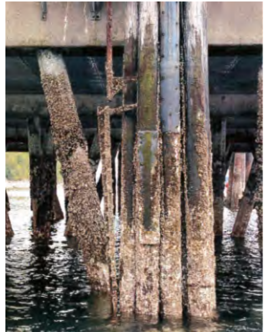
Photo 66: Dolphin D2 with abrasion damage, ladder detached
