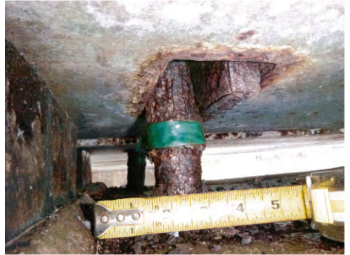
Photo 64: Deck panel 7B hold down bolt is necked down to 1.1875" at pier 7
