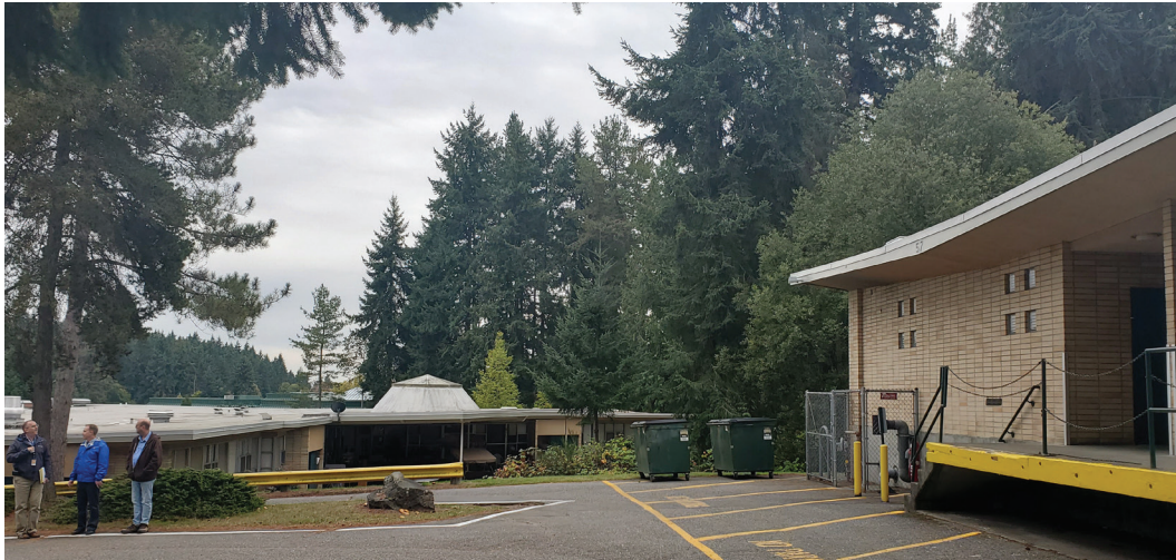
Building Area 1: North
