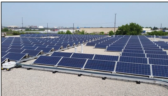
Figure 6: Ballasted racking installation system on flat roof
