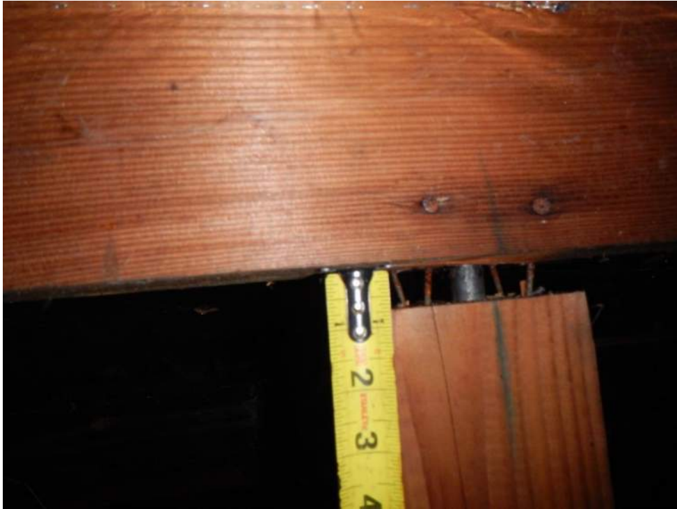
Photograph # 19: High beam separation from post of 3/4 inch.
