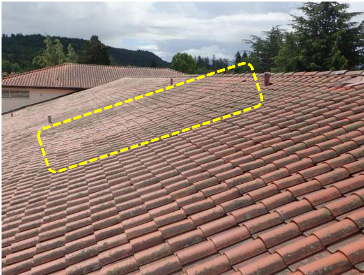
Photo No. 32 - Area of Visual Sagging of Roof Components at Center Wing of Building
