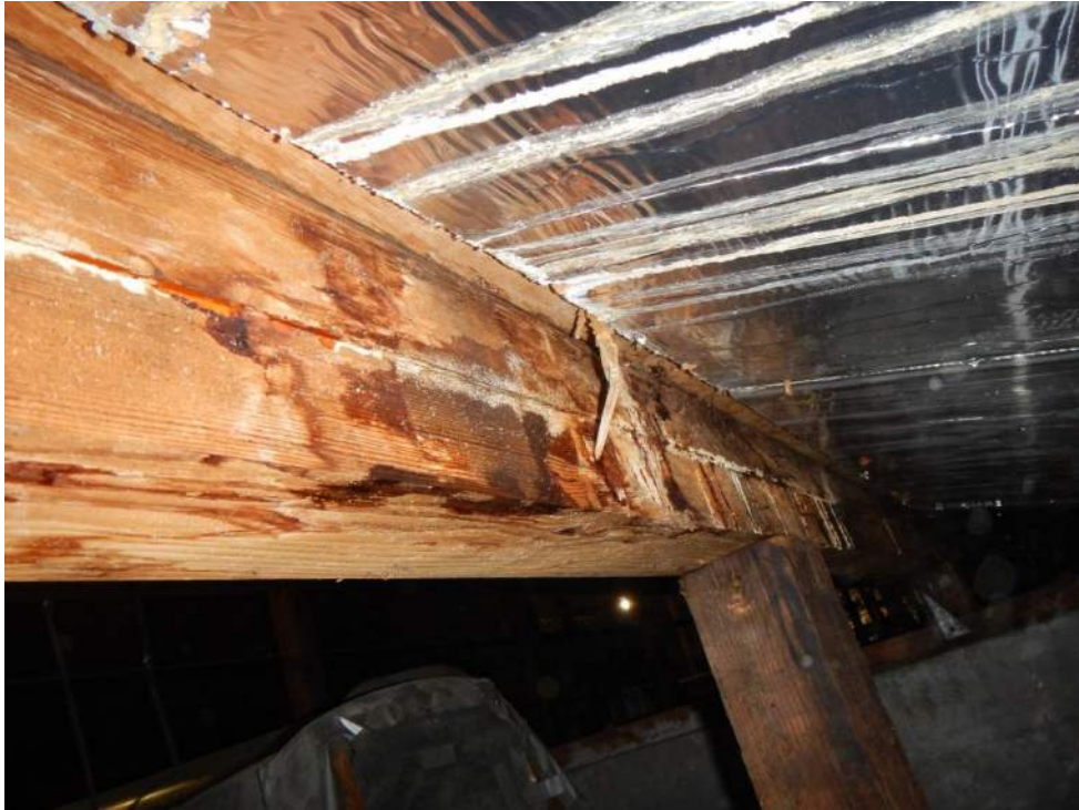
Photograph # 17: Example of seepage staining on soffit of roof decking and support beams.
