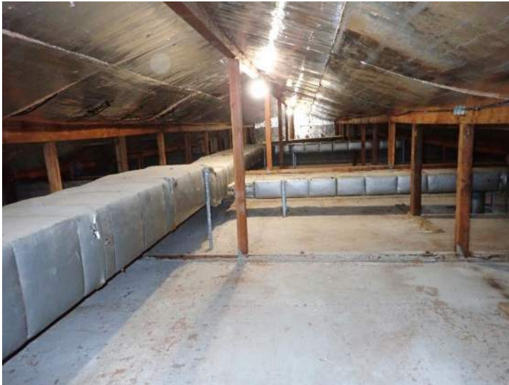
Photo No. 13 - Building 2010 Attic Photo in West Roof Area
