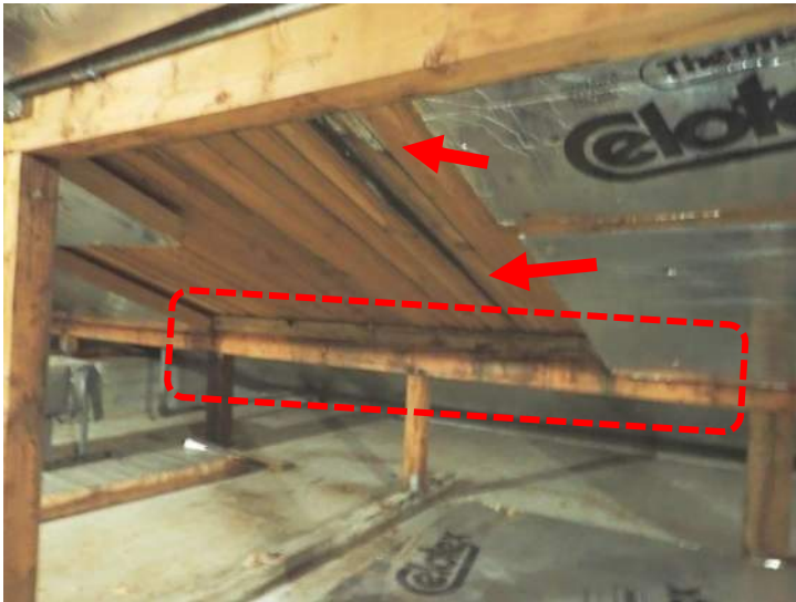
Photo No. 20 - Water Staining at Attic Structural Members
