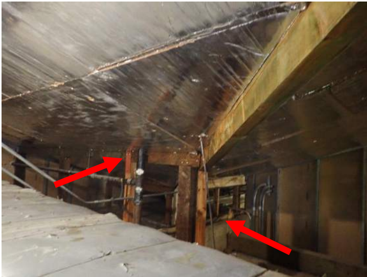
Photo No. 35 - Evidence of Water-Staining at Valleys
