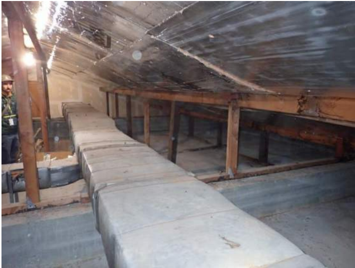
Photo No. 28 - Attic View within West Section of Roof
