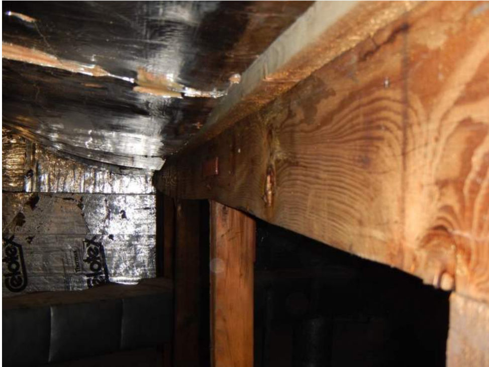
Photograph # 9: Rigid insulation at decking soffit abutting beams and posts.
