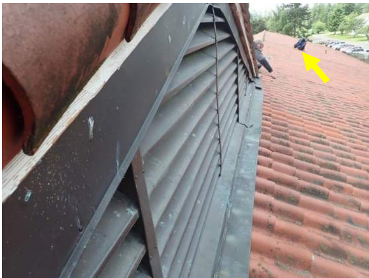
Photo No. 25 - North-facing gable end roof looking west
