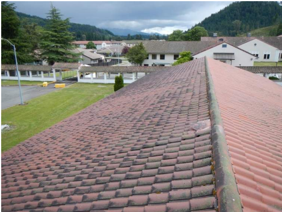
Photograph # 6: View of east roof section of north elevation.
