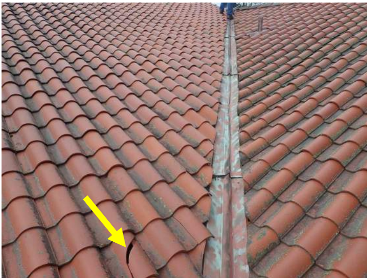
Photo No. 11 - Observations at Typical Valley
