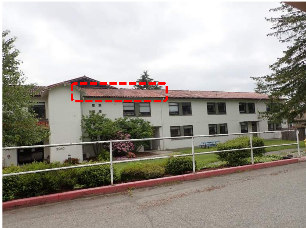
Photo No. 9 - View of the north-facing gable end roof area at the 2010 Building showing the west end of the roof area. It was reported that a portion of the roof area, shown by the red hatched line identified area, was previously repaired to address water-intrusions and water-damaged T&G roof decking.
