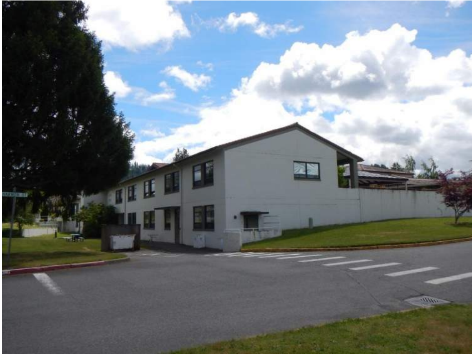
Photograph # 3: View of north-west corner of north elevation.
