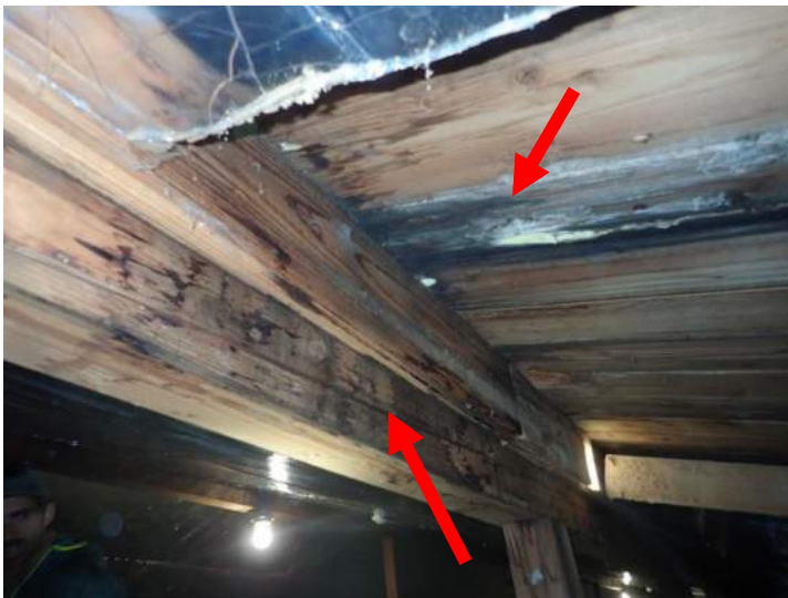
Photo No. 23 - Water Staining and Biological Growth on Wood Structure
