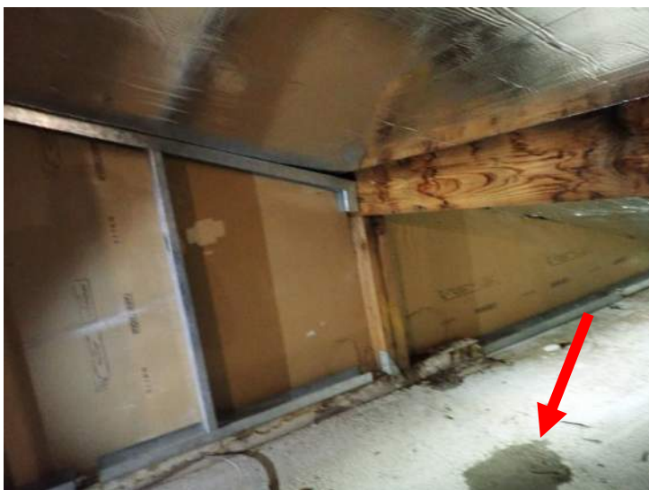
Photo No. 38 - Rain-water leaks Following Brief Storm During Survey
