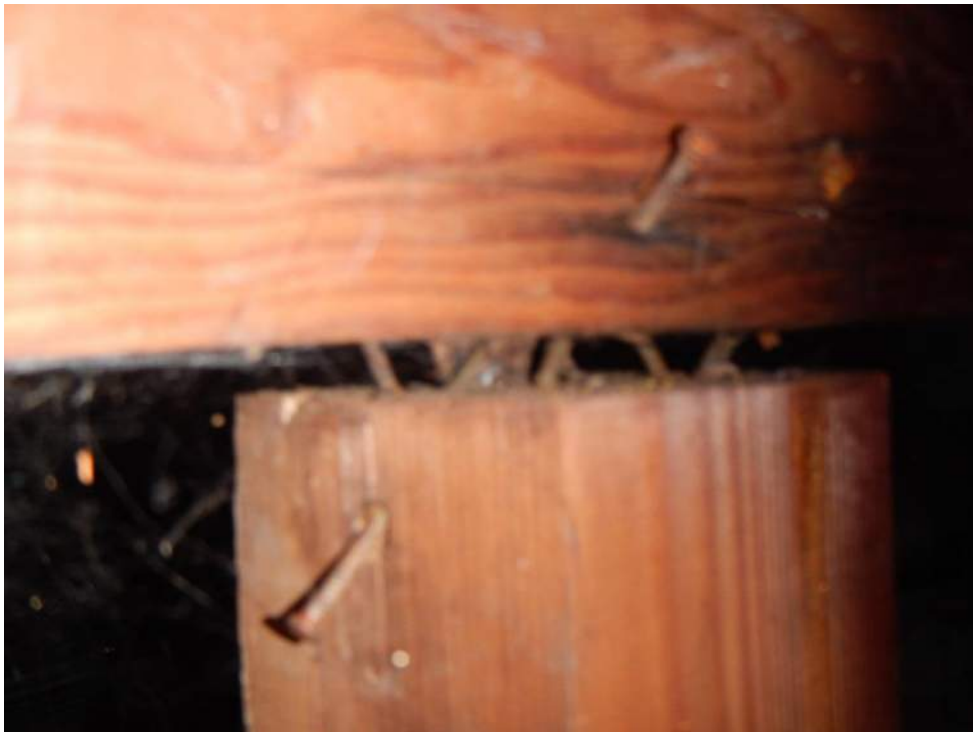
Photograph # 10: Ridge beam not in contact with support post.
