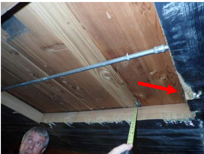
Photo No. 24 - Attic Conditions Downslope from Ridge Vent
