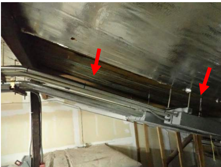
Photo No. 33 - Attic View Below Area of Concern
