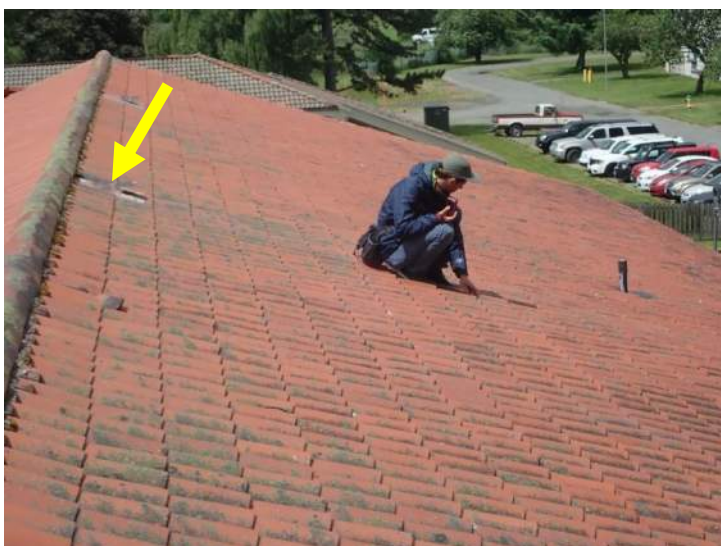
Photo No. 26 - North-facing gable end roof near test area
