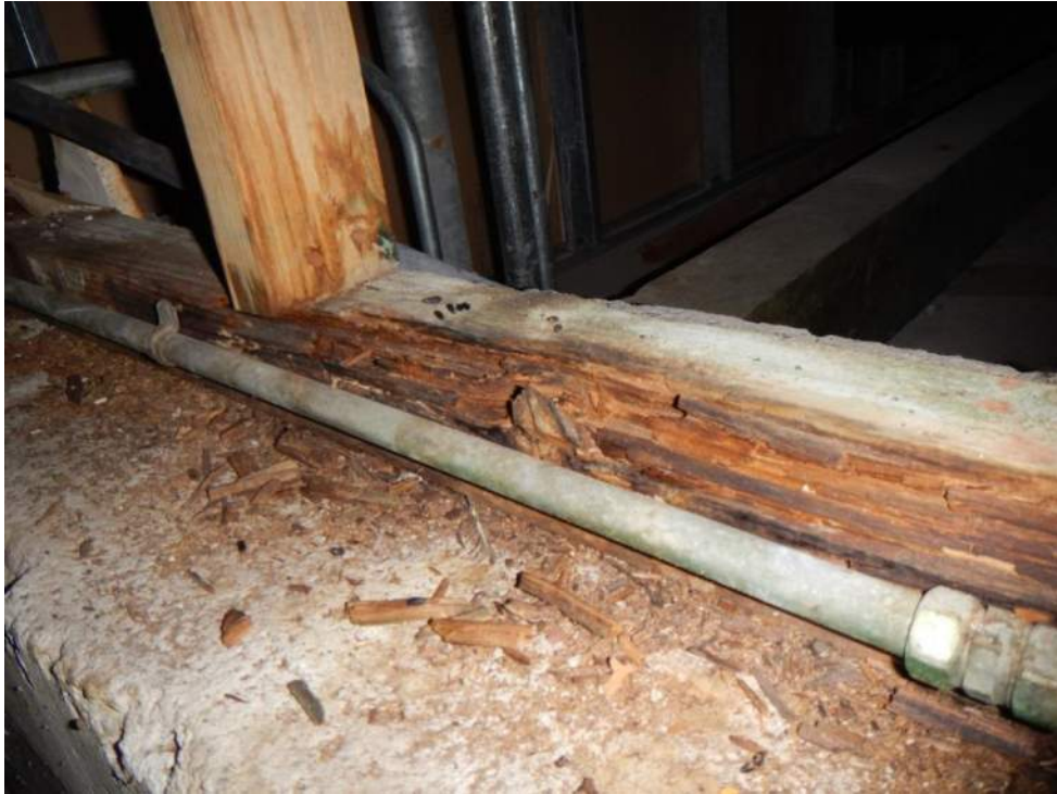
Photograph # 15: Deteriorated wood sill plate below valley on upturned concrete beam.
