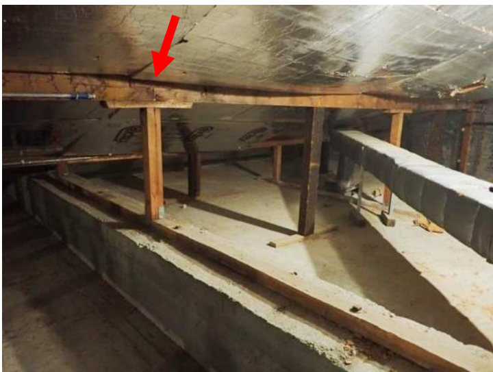
Photo No. 30 - Attic View within East Section of Roof
