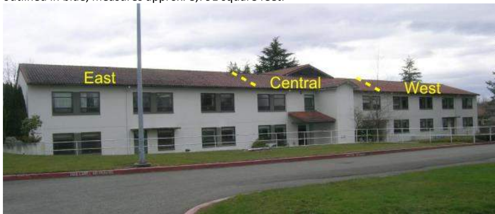
Photo No. 7 - View of the north-facing gable end roof area at the 2010 Building that was the primary focus of our roofing survey. Area separation walls built within the attic break the space into sections identified here as East, central, and West, as indicated in this photo.
