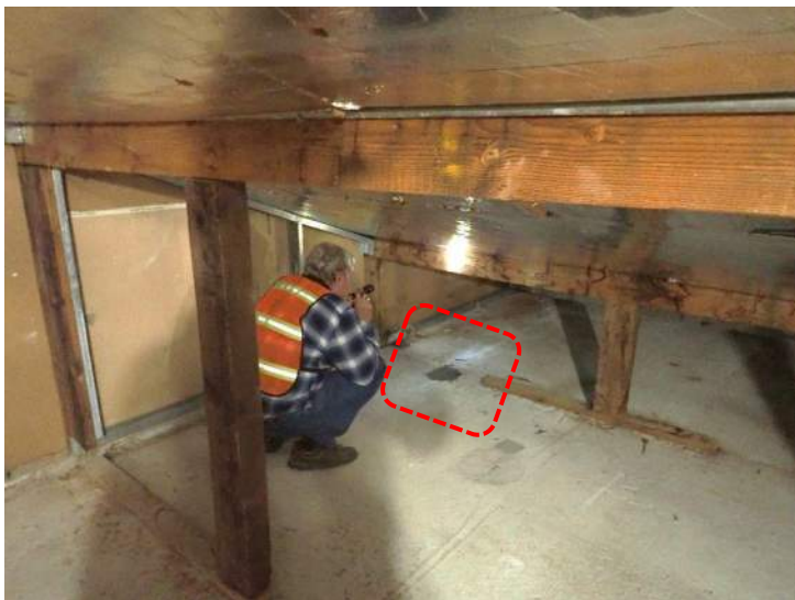
Photo No. 37 - Rain-water leaks Following Brief Storm During Survey
