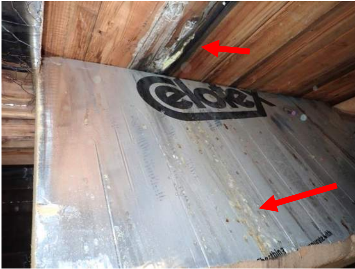
Photo No. 22 - Water Staining and Biological Growth Trapped by Insulation
