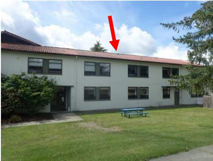
Photo No. 16 - Building 2010 North End Roof Area
