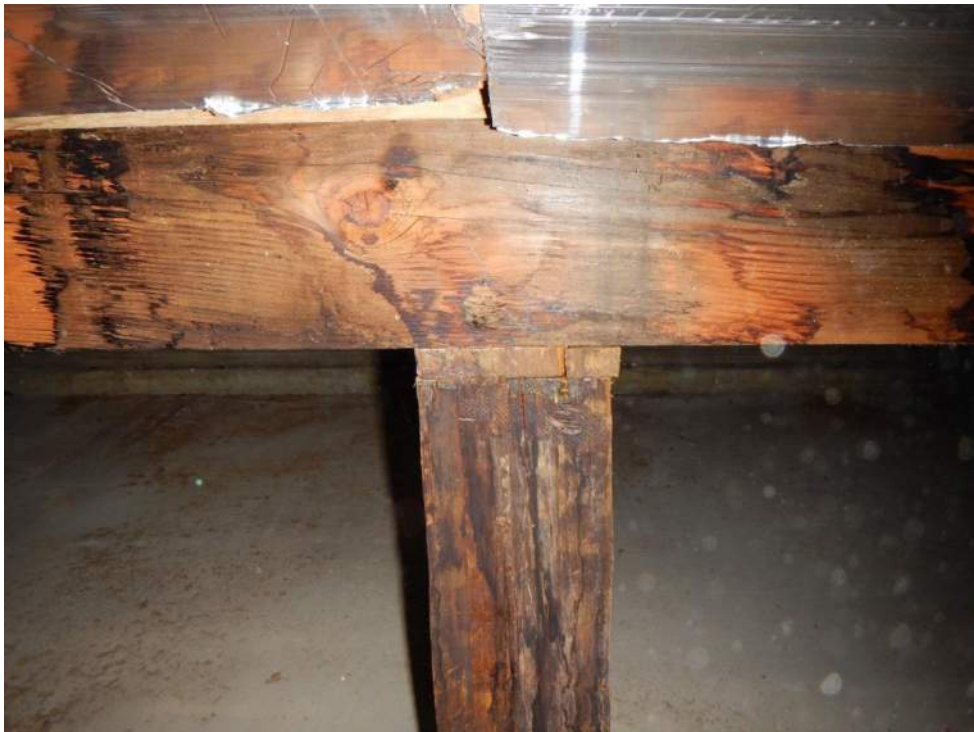
Photograph # 8: Example of water seepage staining on beam and post.
