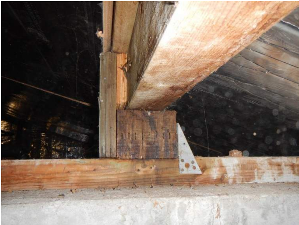
Photograph # 18: Repair of short timber post on upturned concrete beam.
