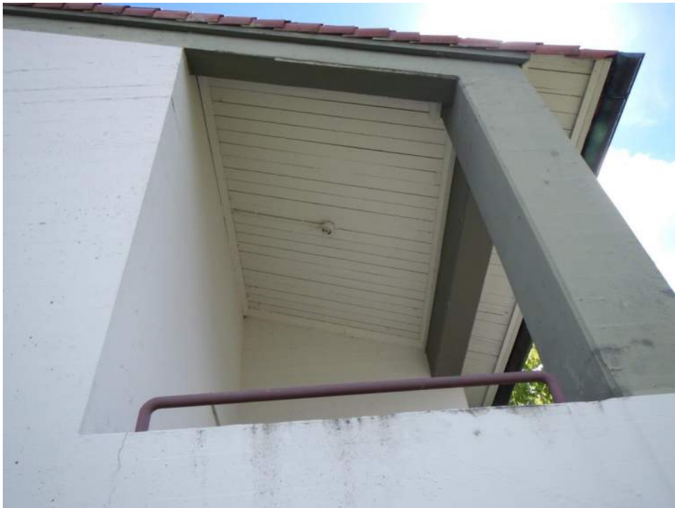
Photograph # 4: Exposed roof decking at corner porch recesses.
