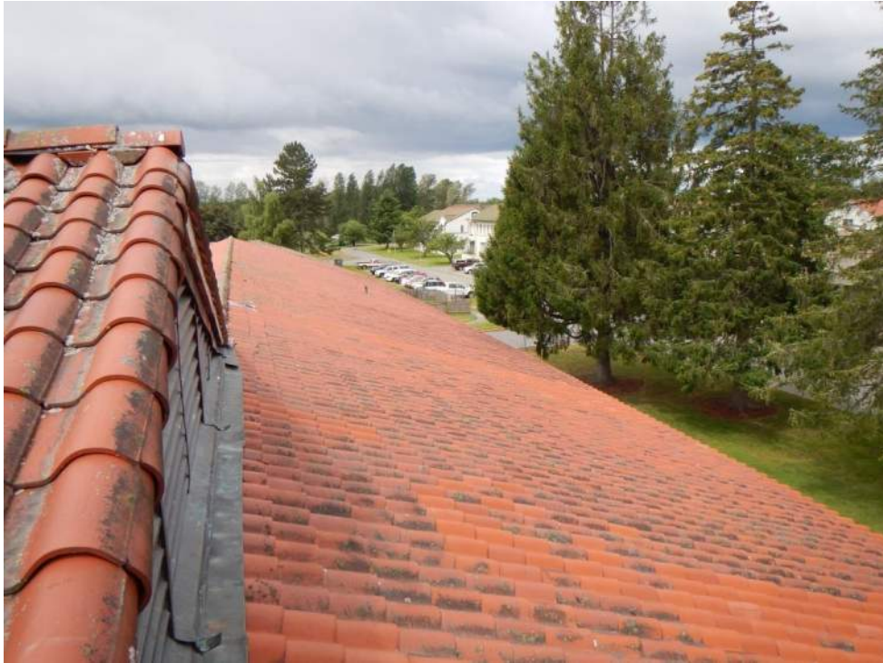
Photograph # 5: View of west roof section of north elevation.
