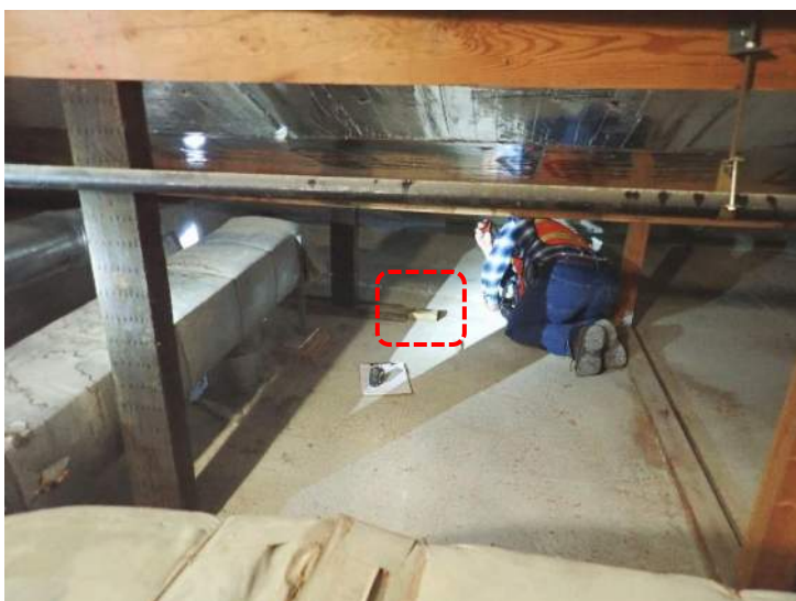
Photo No. 39 - Rain-water leaks Following Brief Storm During Survey
