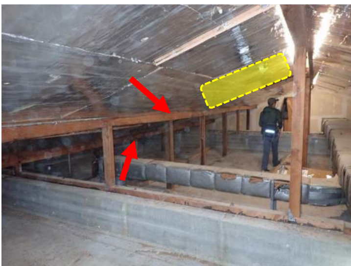
Photo No. 15 - Building 2010 Attic Photo in West Roof Area
