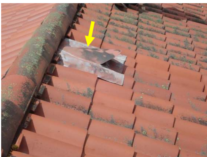
Photo No. 27 - Example gable vent at north end roof area
