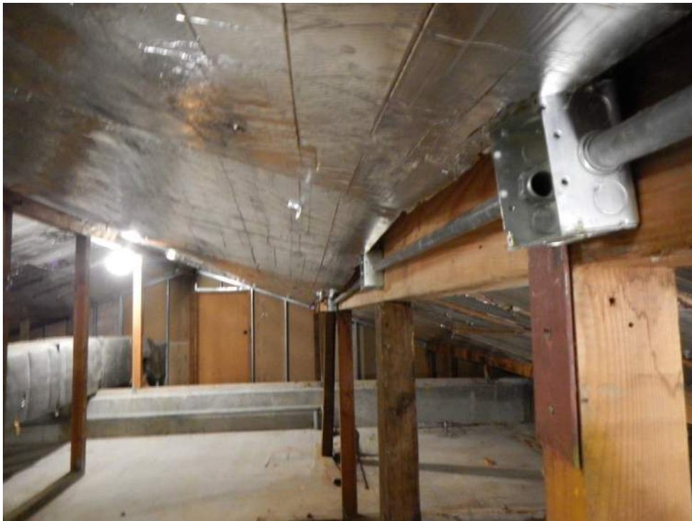
Photograph # 14: View of attic framing with rigid insulation (note non-plumb posts)
