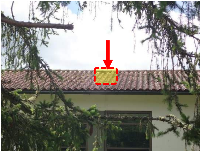
Photo No. 17 - North End Roof Area and Ridge Vent at Test Area
