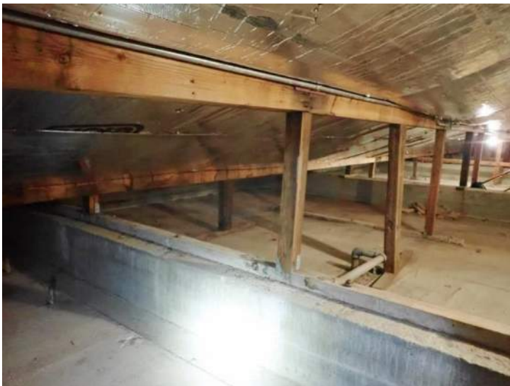
Photo No. 29 - Attic View within Central Section of Roof
