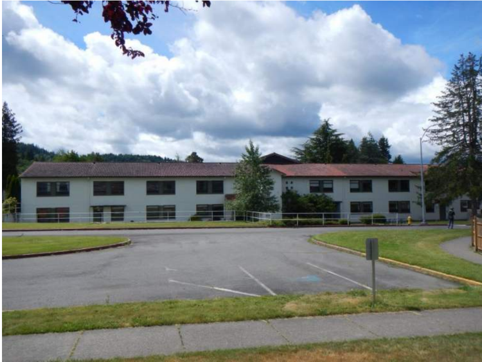
Photograph # 1: Overall view of building north elevation.
