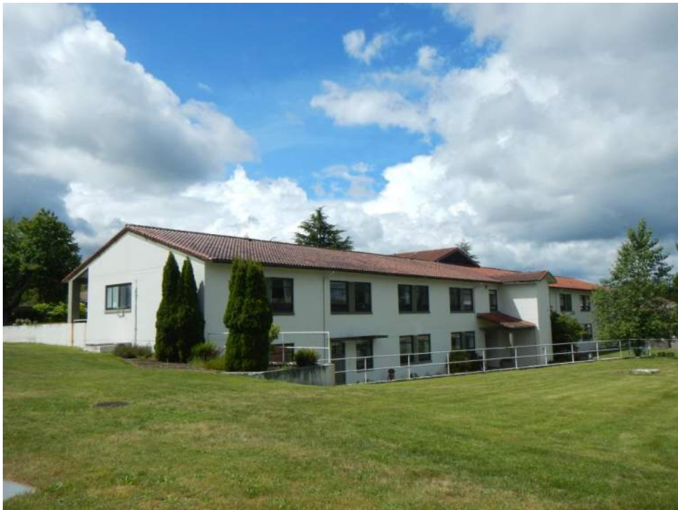
Photograph # 2: View of north-east corner of north elevation.
