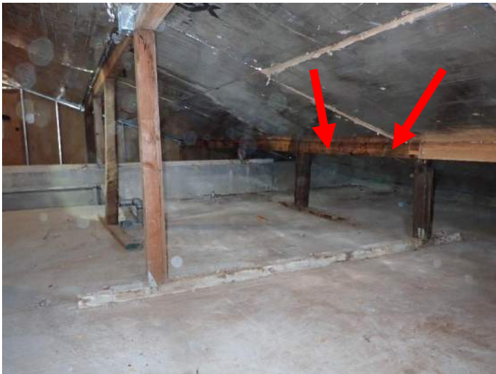
Photo No. 14 - Building 2010 Attic Photo in Center Roof Area
