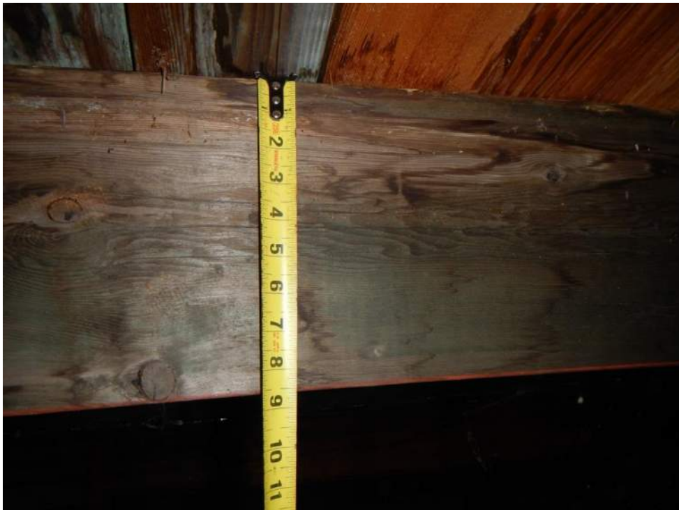
Photograph # 16: Example of plumb shaped 4X roof support beam.
