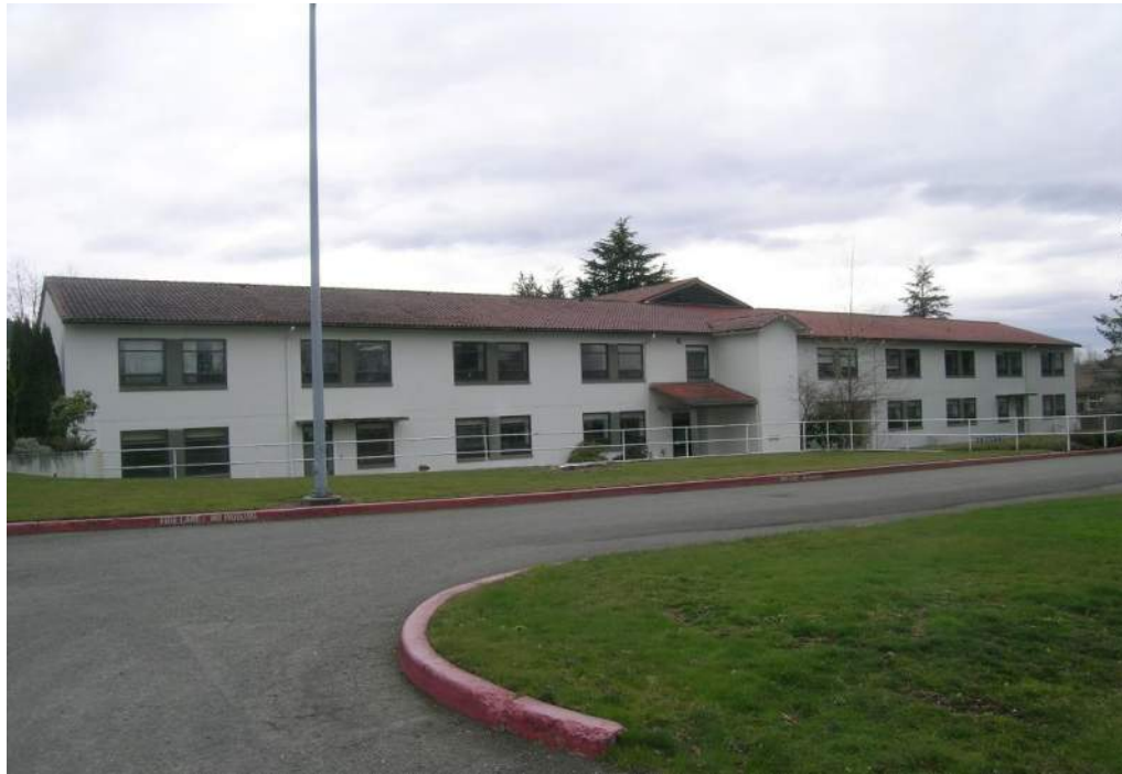
Photo No. 8 - View of the north-facing gable roof area at the 2010 Building that was the primary focus of our roofing survey.
