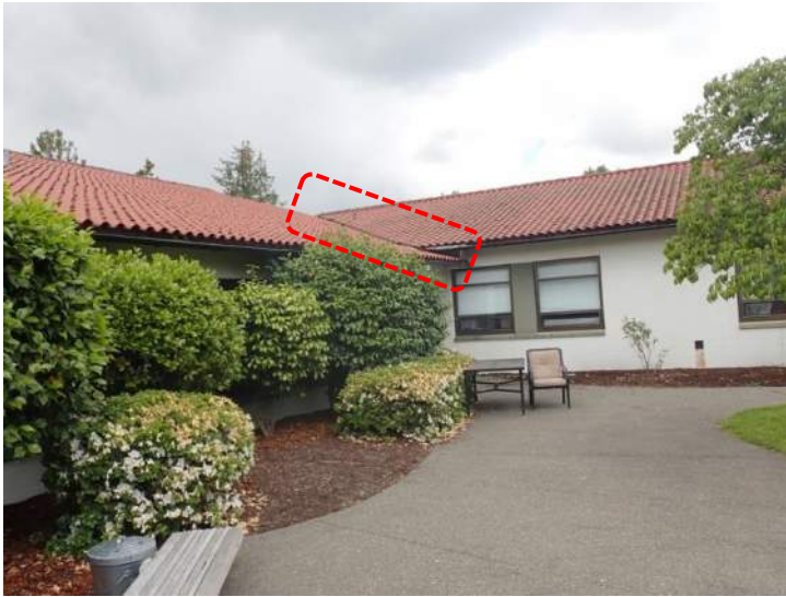
Photo No. 34 - Valley at East Side of Roof Survey Area
