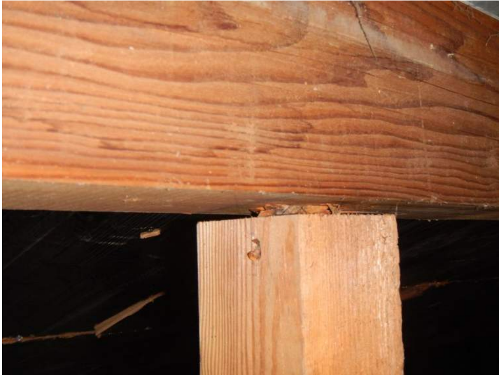
Photograph # 13: Ridge beam not in contact with support post.
