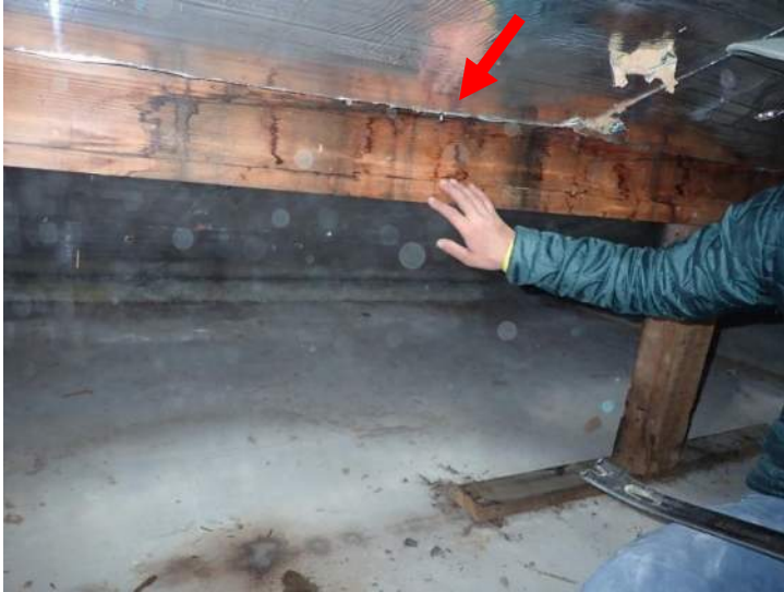
Photo No. 19 - Systemic Water Staining at Attic Wood Beams
