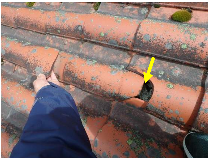
Photo No. 12 - Example of Cracked and Broken Roof Tiles Observed in Field of the Roof Areas
