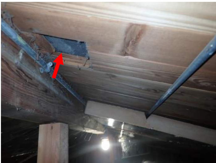
Photo No. 18 - Attic view at Ridge Vent Location
