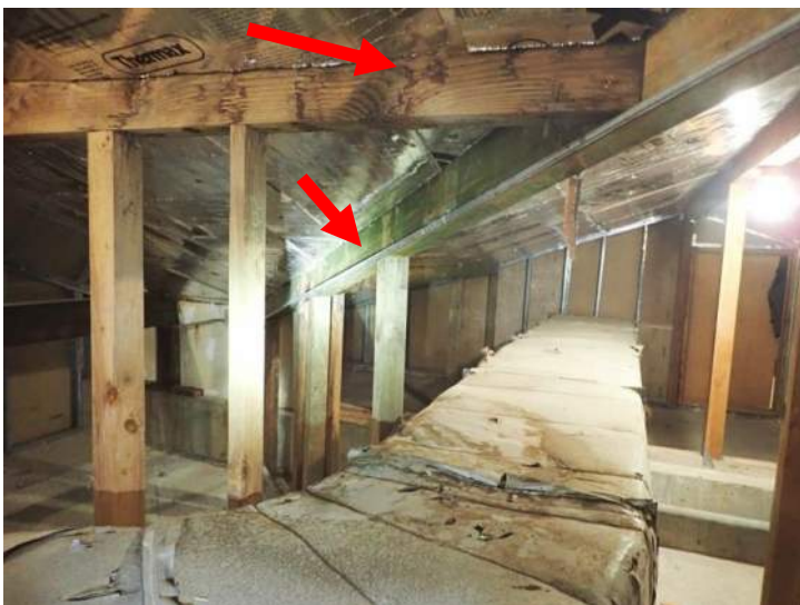
Photo No. 36 - Evidence of Water-Staining at Valleys
