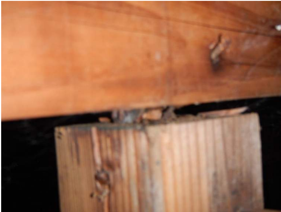
Photograph # 11: Ridge beam not in contact with support post.
