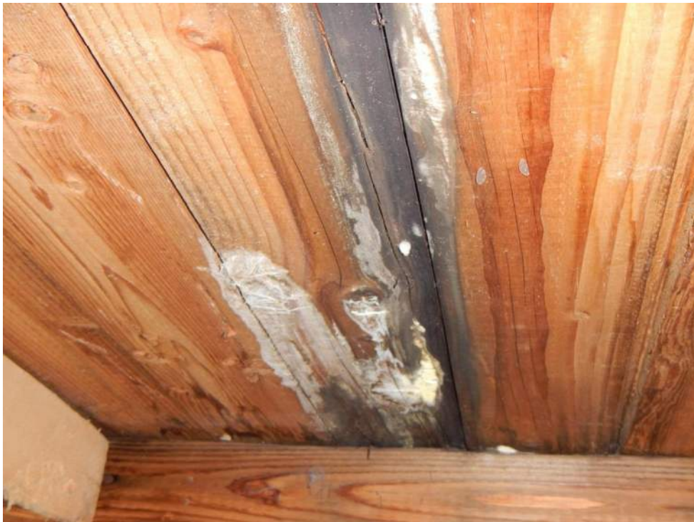
Photograph # 12: Example of timber roof deck decay at soffit.
