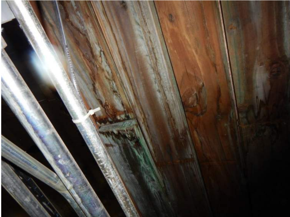
Photograph # 7: Example for water seepage staining on soffit of decking.
