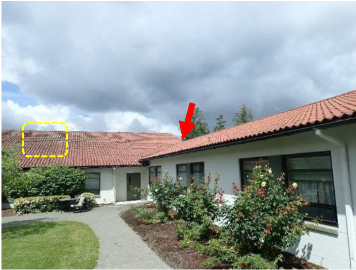
Photo No. 31 - East Courtyard showing Valley at Area of Concern
