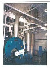
Installation of a DC-2-500 SUPERMIZER servicing a 500 H.P. boiler.
