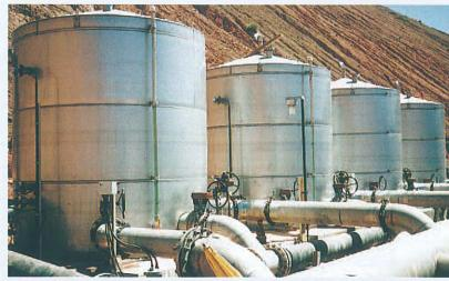
Four of sixteen 12,000 gallon T-316L stainless steel tanks for acidic leach solution in mining operations for Bechtel Corp.
