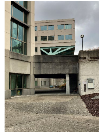
Pass under a walkway.
